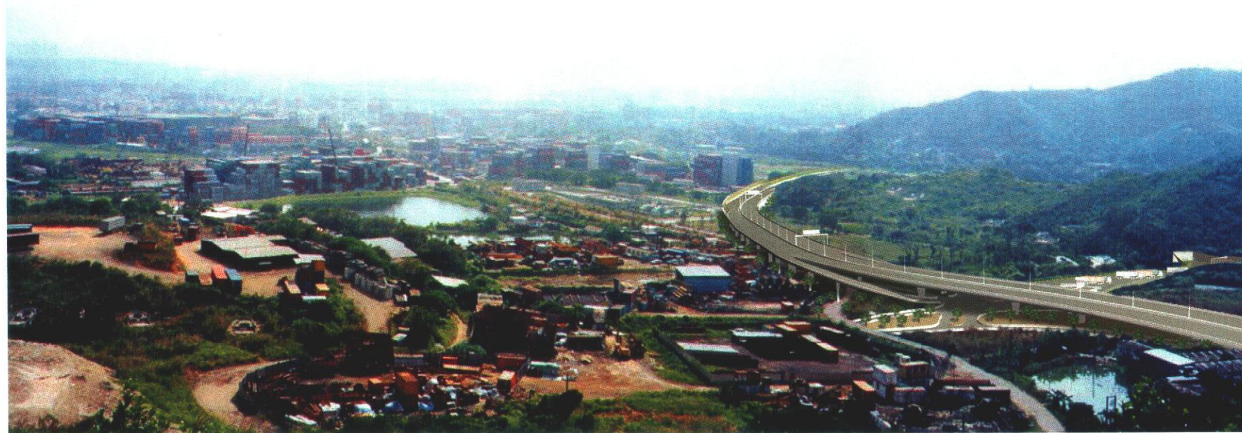
Photo View No. 7.3 Viewed from Hill North of San Wai - Day 1 With Mitigation
