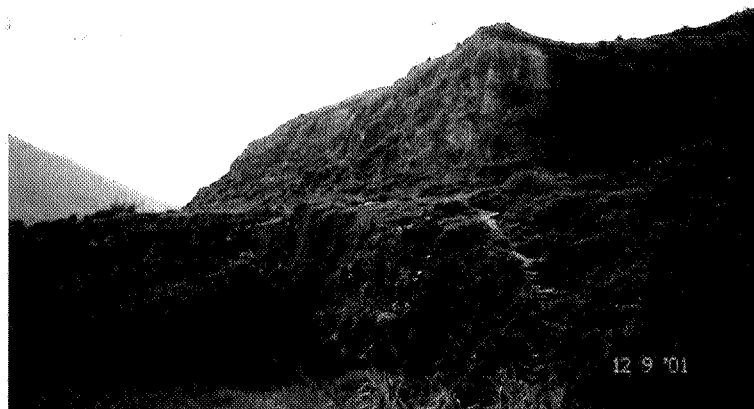
Patches of low scrub/grass growing on exposed slope north of the shipyard due for reprofiling work
