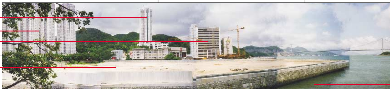
VIEW TAKEN FROM LIDO GARDEN - FACING THE RIDGE LINE OF TAI MO SHAN TO THE EAST
