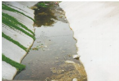
River channel has been strengthened with shotcrete and the existing water quality is poor with algal mat attached on rocks. The naturalness and diversity of the stream is greatly reduced.
