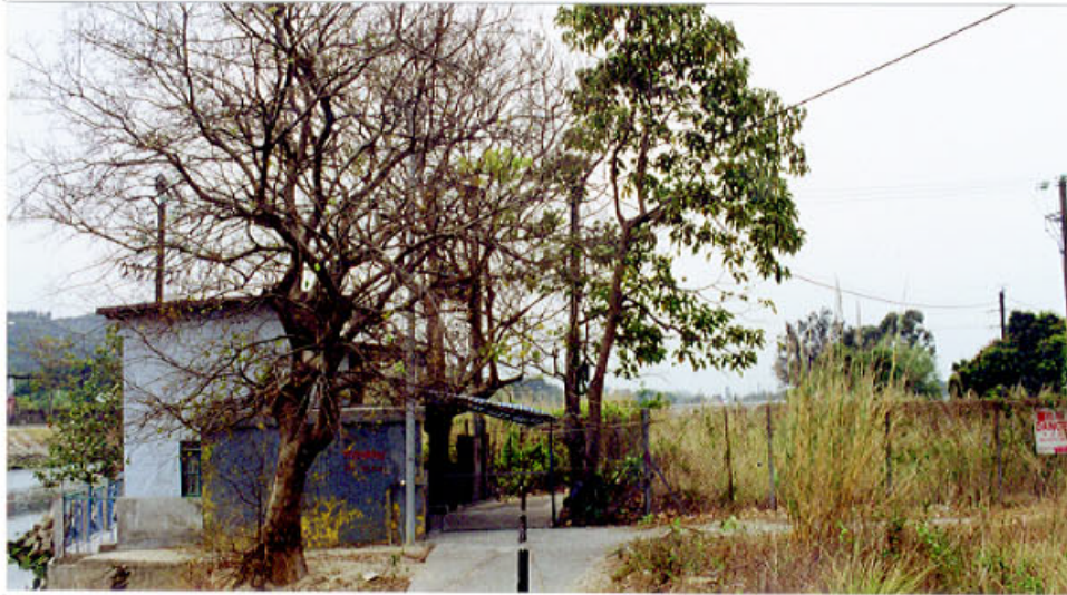
Photograph A CARE REQUIRED TO ENSURE SEWER ALIGNMENT AVOIDS MATURE TREES
