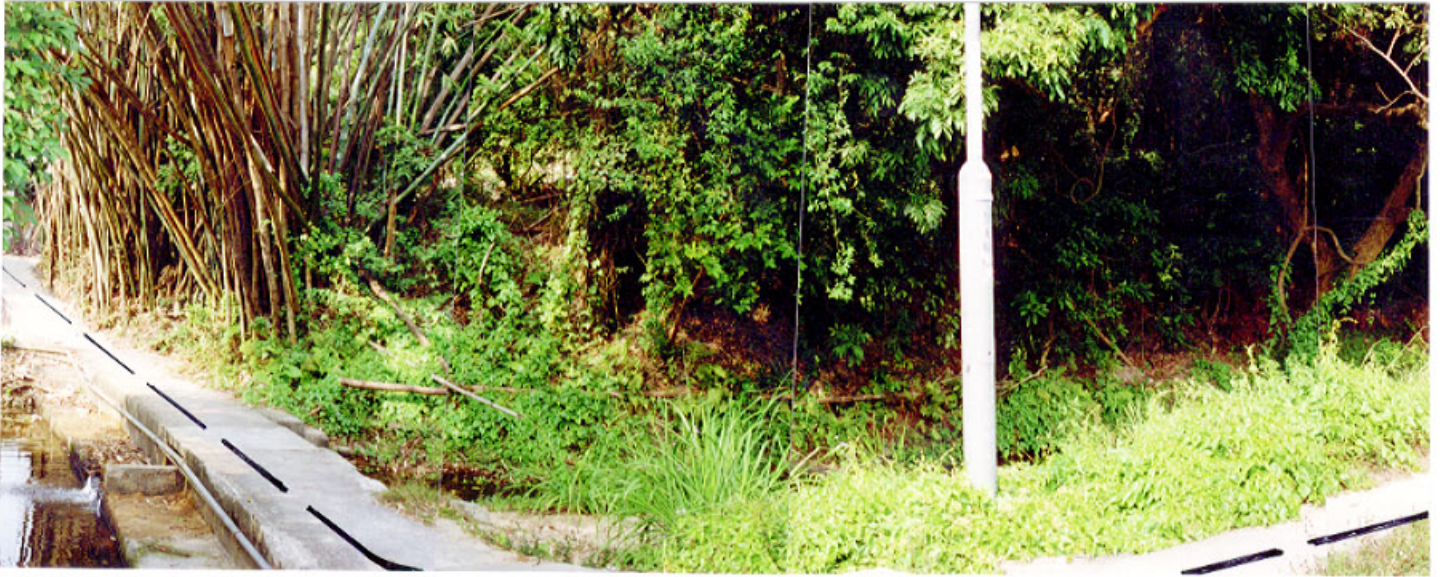
Photograph A ADOPTED REALIGNMENT OF SEWER TO AVOID WOODLAND FRINGE AND FOLLOW EXISTING CONCRETE TRACK (REFER DWG. 10.3)
