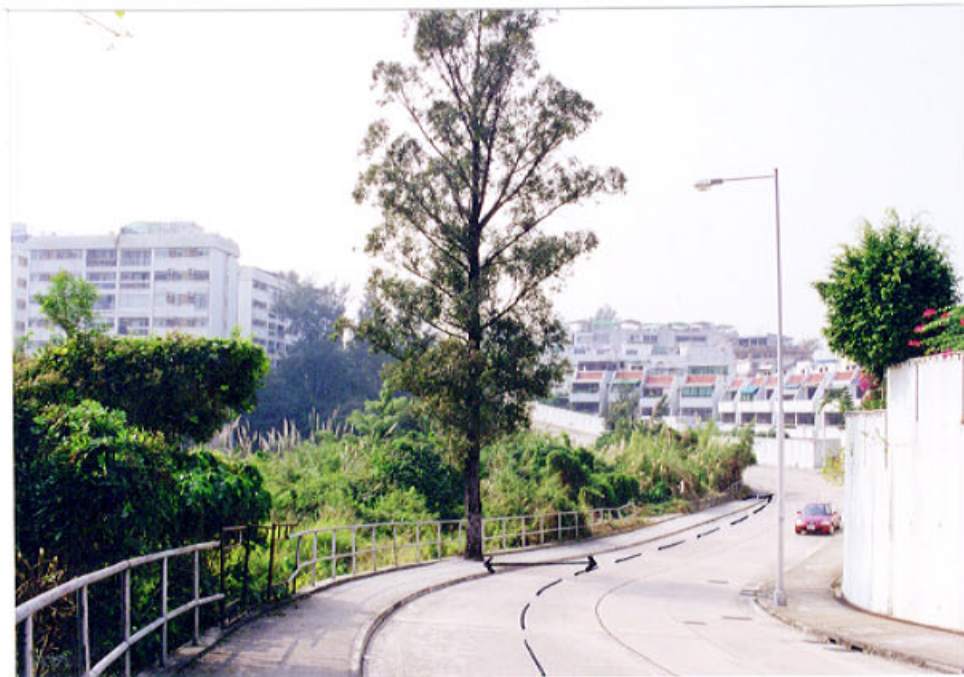
Photograph B RECOMMENDED REALIGNMENT OF SEWER INTO STREET TO AVOID DAMAGING ROOTBALL OF MATURE ROADSIDE TREE
