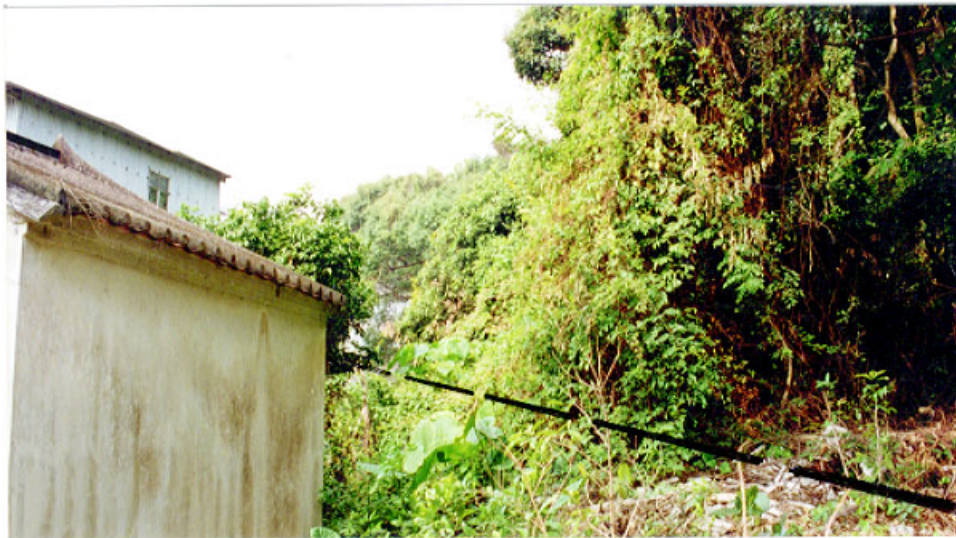
ORIGINAL SEWER ALIGNMENT BEHIND WONG UK VILLAGE RELOCATED INTO PARALLEL VILLAGE LANE AS RECOMMENDED TO AVOID TREE FELLING (REFER DWG. 10.2)
