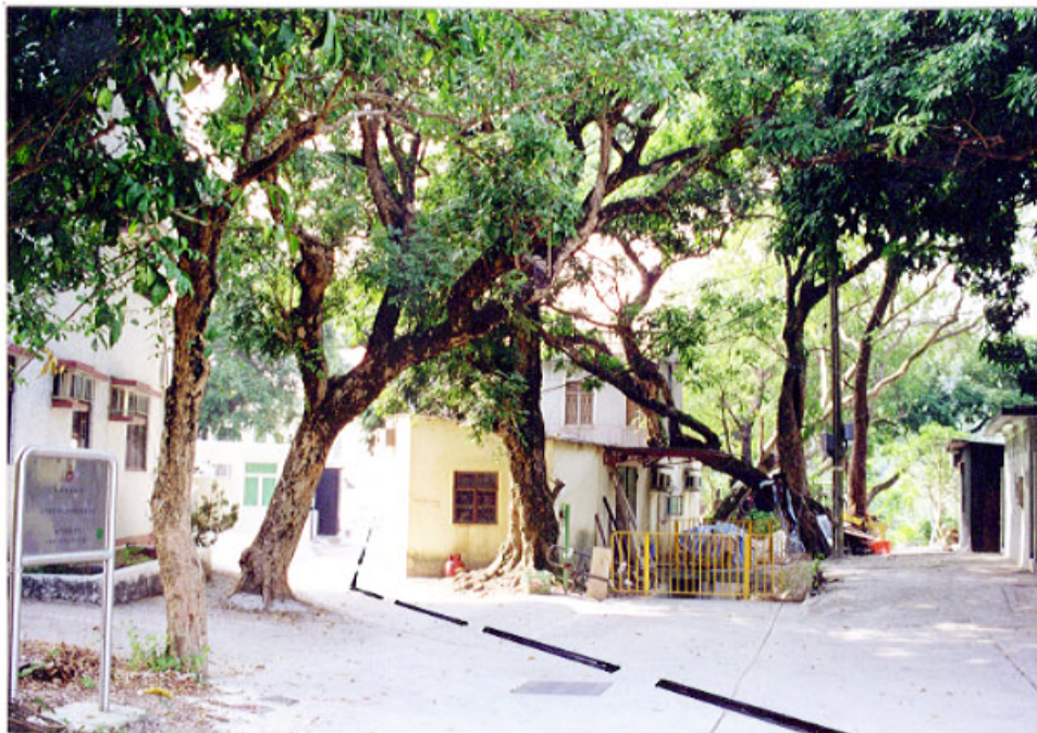
Photograph B CARE REQUIRED WITHIN VILLAGE TO ENSURE SEWER AVOIDS MATURE TREES IN NARROW LANES
