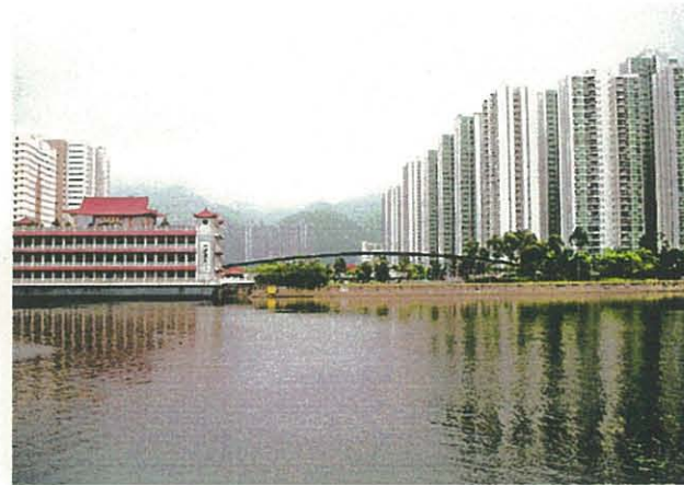
Figure 7.6E View from Rowing Centre directly opposite proposed flyover partly screened by east bank promenade trees
