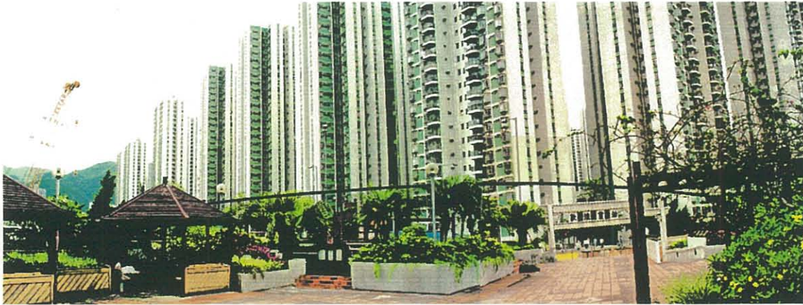
Figure 7.9 View from Floating Restaurant Garden and Playground. Flyover is located immediately behind entrance gate
