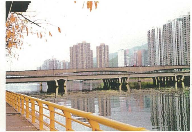
Figure 7.6C Sha Tin and Fo Tan Road bridges block views from southern portion of west bank promenade
