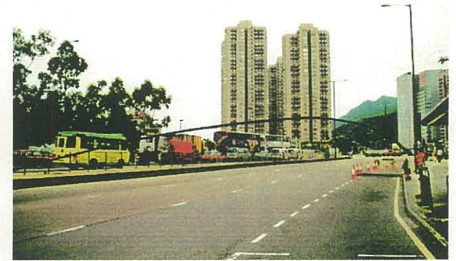
Figure 7.8D View north along Tai Chung Kiu Road from City One Estate towards flyover junction
