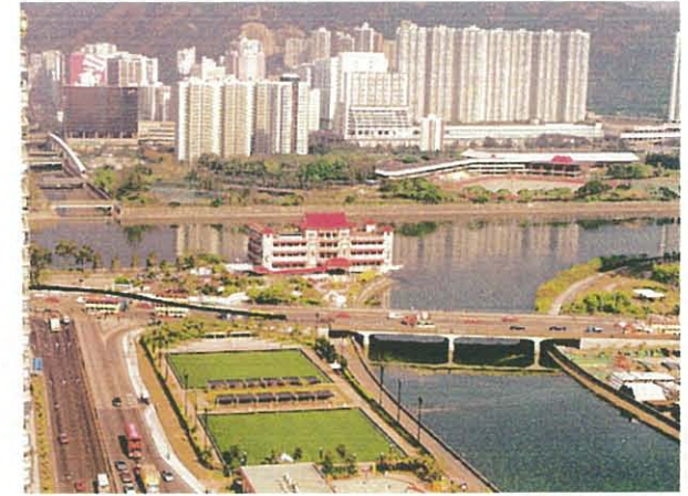
Figure 7.10 View from top floor of City One Estate residential block
