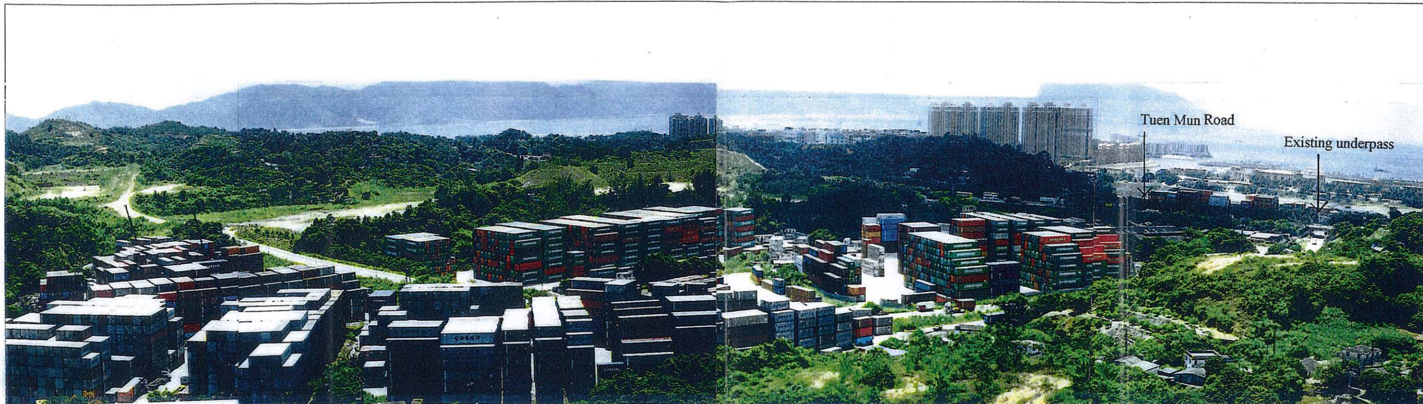
VIEW SHOWING THE EXISTING LANDSCAPING
