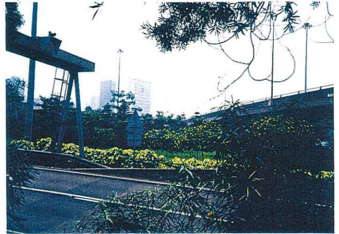
Photograph 10 Amenity planting adjacent to the Eastern Harbour Crossing Tunnel Entrance.
