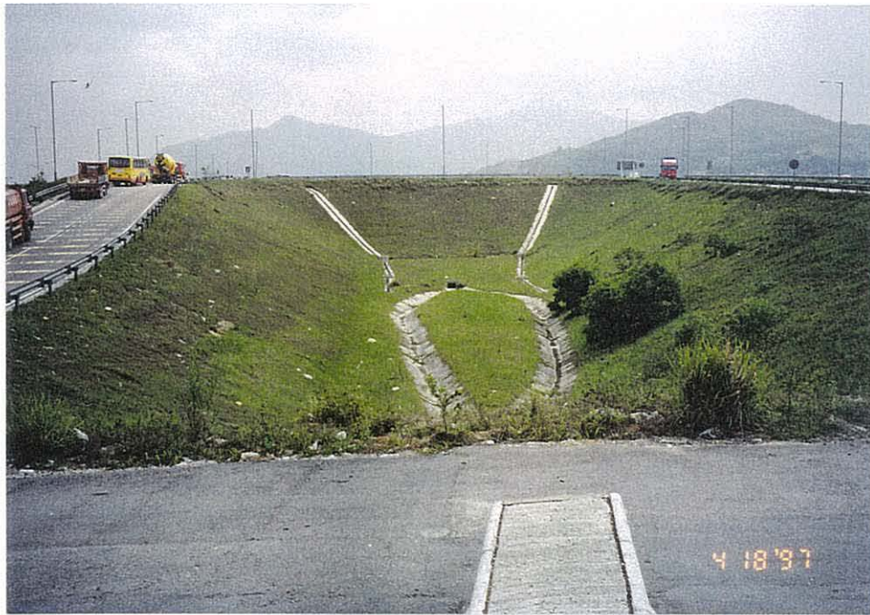
Photo 8. Southern side of Shak Pat Heung Interchange. The shrub on the lower right corner were young Acacia confusa . (View: south to north, location 7)
