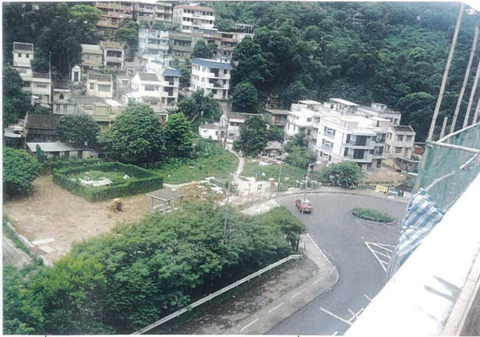
Low Value Wasteland and Marsh at base of Lok Lo Ha Village Existing Access Road
