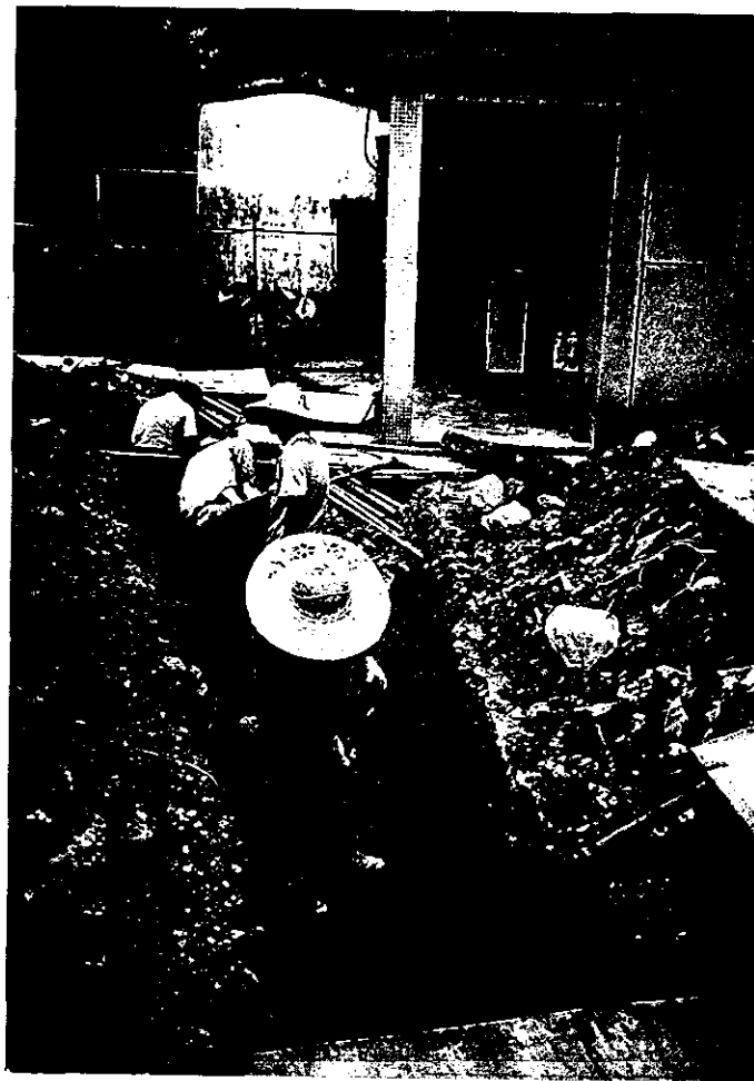
Figure C-1-1: Excavation Works for Village Sewerage - Stage I Phase I
