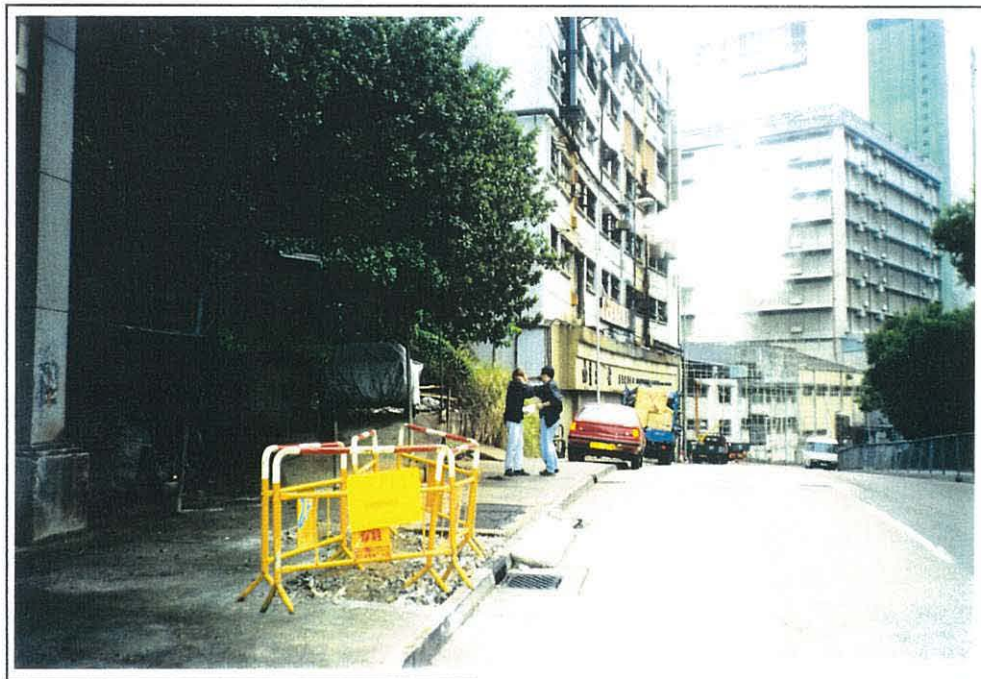
Plate 7.3 Site of Proposed Sewer Connection - Tsuen Wan WTW
