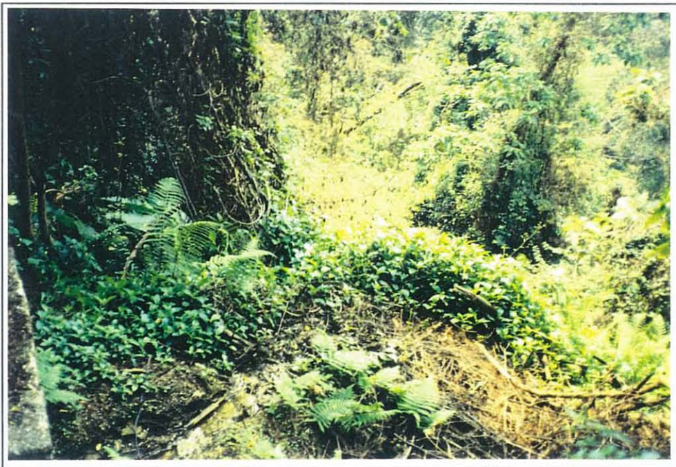
Plate 12.5 Slope Below Mouth of Sludge Disposal Pipe - Tai O
