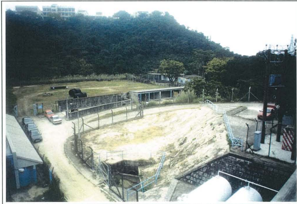
Plate 9.2 Site for Proposed Wastewater Recovery Tanks - Tai Po Road WTW
