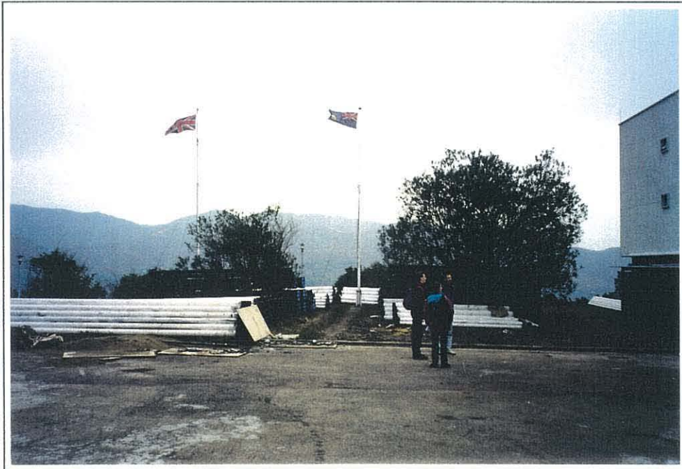
Plate 11.2 Site for Proposed Dewatering House - Silvermine Bay WTW
