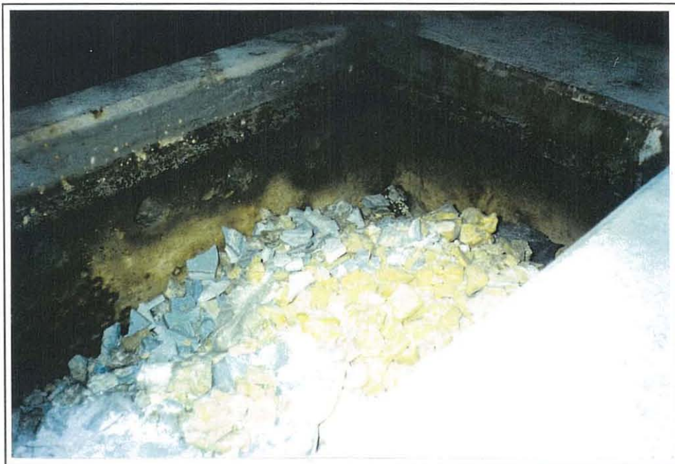
Plate 2.2 Lime powder stored prior to addition to raw water.
