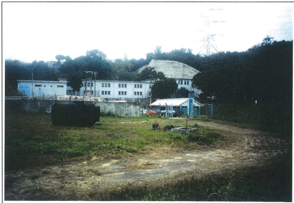
Plate 9.3 Site for Proposed Wastewater Recovery Tanks - Tai Po Road WTW
