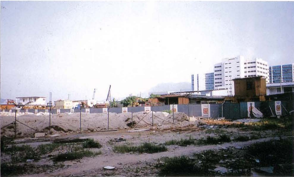
View South over East Kowloon Reclamation Site
