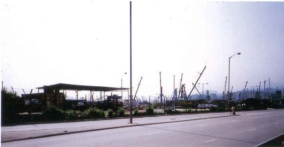
View to the North along Ferry Street and Proposed West Kowloon Reclamation Site
