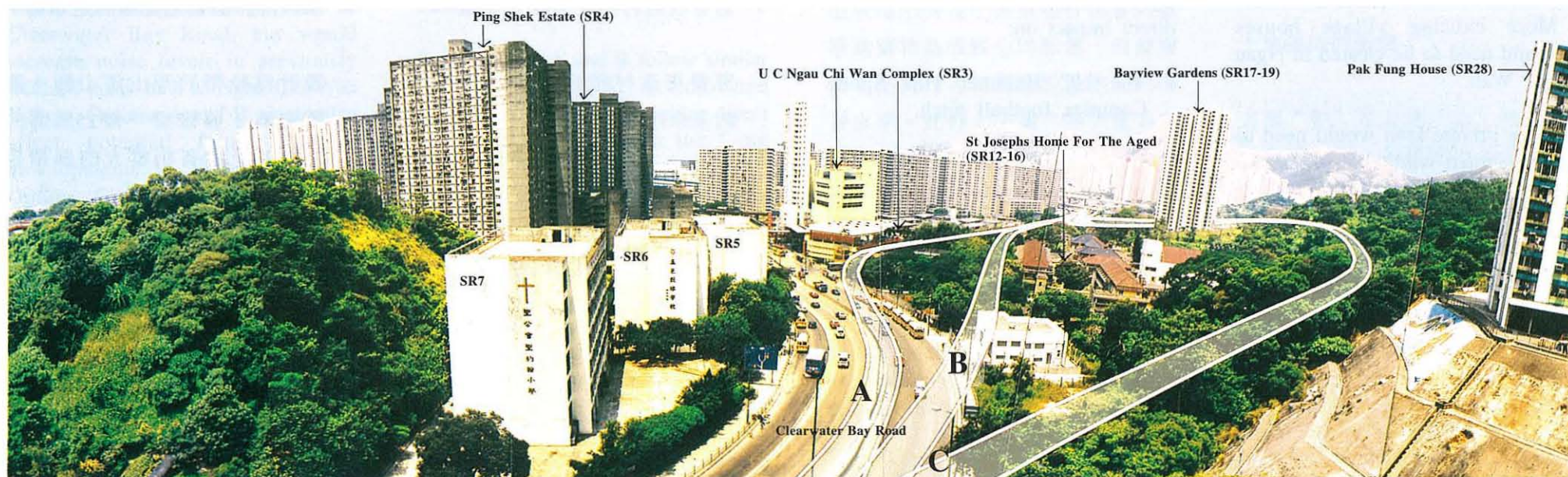
Figure 5 - View 2: From Roof Top of Choi Wan St Joseph's Primary School (SR11)
