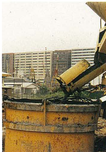
PFA is mandatory in concrete for roads. 煤灰粉是道路混凝土必不可少材料 Placing PFA concrete in pile heartings. 橋中澆築煤灰粉混凝土
