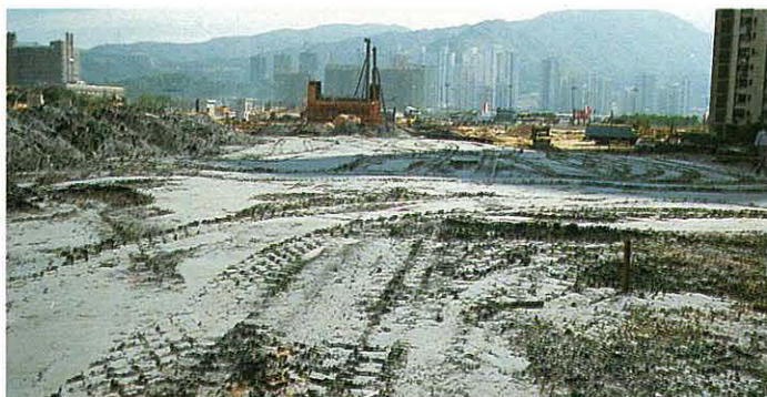
Placing PFA fill in the embankments. 澆築橋台煤灰填層
