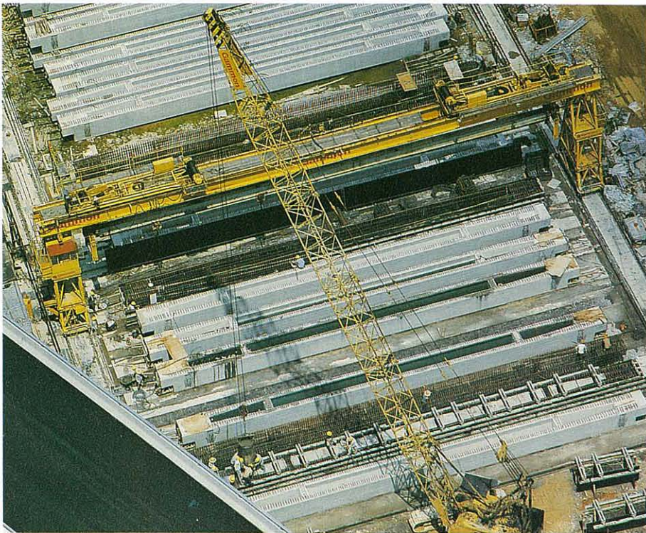
The precast beam fabrication yard. 預先安裝橫樑場地。
