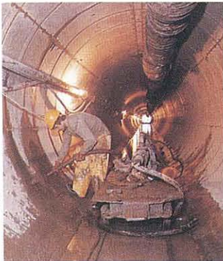
Tunnel grouting with PFA. 煤灰漿築隧道
