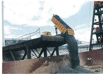
Loading conditioned PFA into barges. 煤灰濕料裝(駁)船
