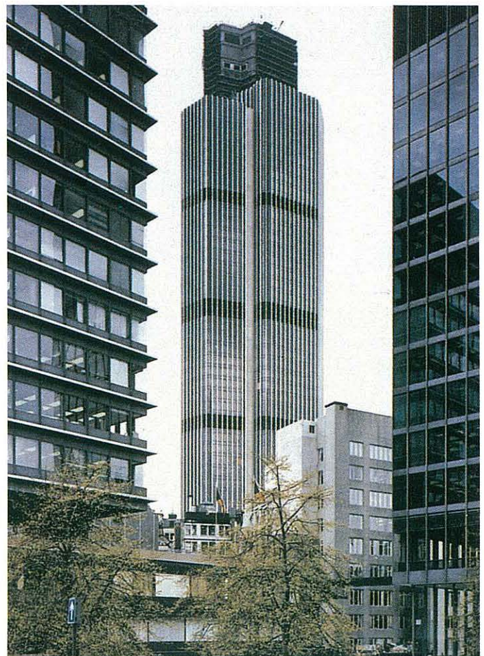
The National Westminster Tower, London, used lightweight PFA aggregate. 倫敦輕質骨料建築的英國西敏銀行大廈
