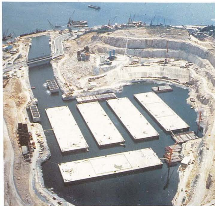
Tunnel units being floated out for placing. 隧道段浮起及拖運
