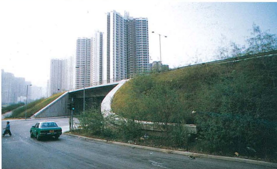
Contract TM 33/84 used PFA fill for highway embankments. The buildings behind are built over PFA fill. TM 33/84號合約煤灰填築公路路堤。堤後建築物均建於煤灰填地上。
