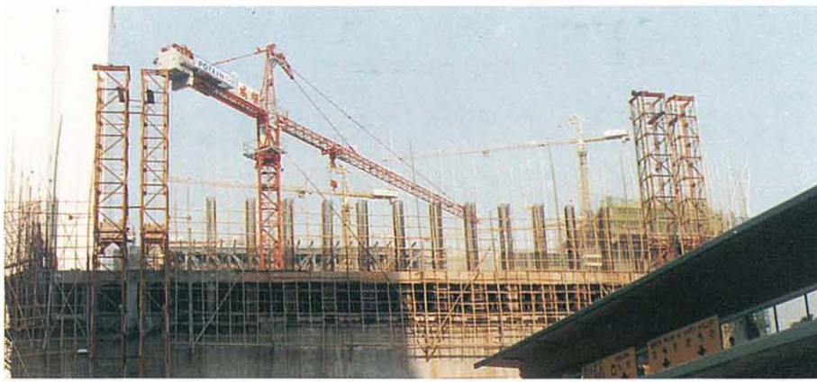
Early stages of construction. 早期施工景象
