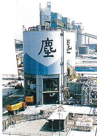
The PFA silos at the Castle Peak Power Stations. 青山電廠煤灰粉倉
