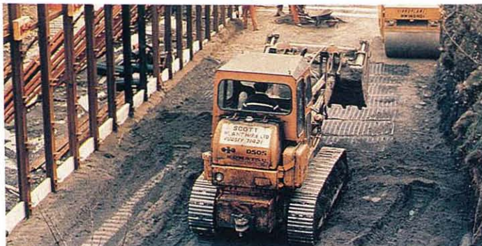
PFA and polymer grids for reinforced soil applications. 煤灰及塑膠網強化土壤
