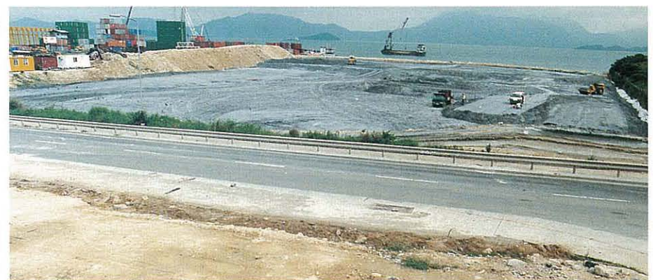
General view of Area 47S showing compaction trials in progress. 47S 區全景
