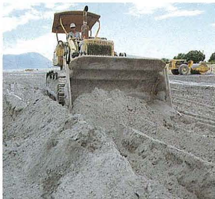
Spreading and placing PFA. 煤灰鋪整情況
