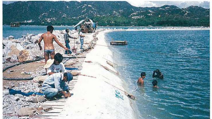
Construction of a PFA concrete watertight membrane. 煤灰混凝土築隔水牆
