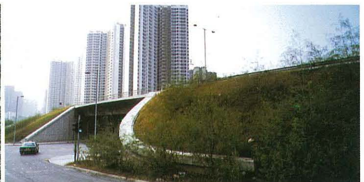
The completed embankment after grassing. 路堤竣工鋪草後全景
