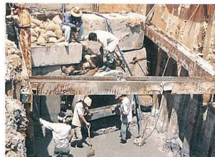
Trenching through the PFA. 煤灰層掘溝
