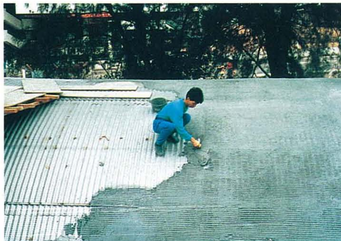
Refurbishment of army huts with PFA mortar. 用煤灰漿翻修軍隊營房
