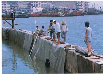
Placing geotextile filter membrane. 鋪設濾膜布層
