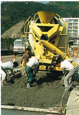
PFA is mandatory in concrete for roads. 煤灰粉是道路混凝土必不可少材料 Placing PFA concrete in pile heartings. 橋中澆築煤灰粉混凝土
