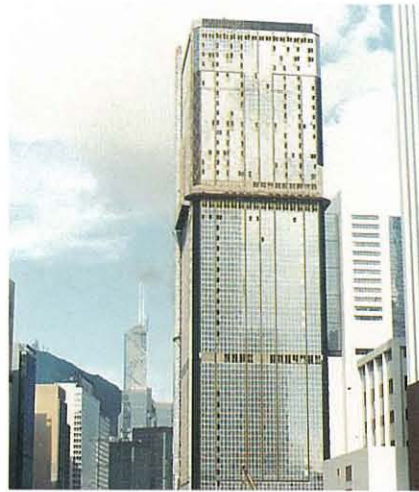
Building nearing completion. 合署接近竣工全景
