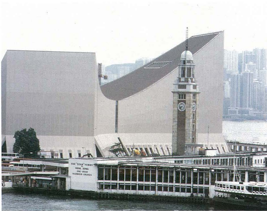
The completed Cultural Centre. 文化中心竣工全景
