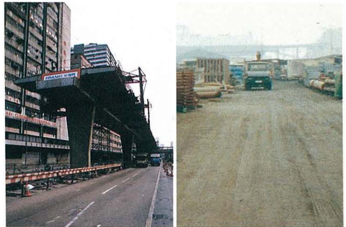
PFA concrete in elevated highway structure.
