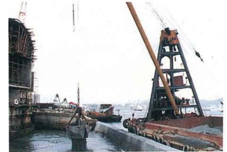
Placing PFA in reclamation. 煤灰填海
