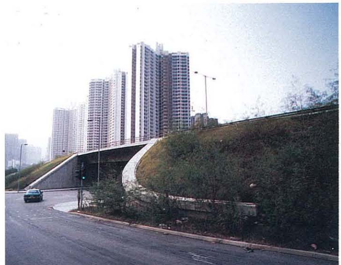
PFA road embankment in Tuen Mun. 屯門煤灰路堤
