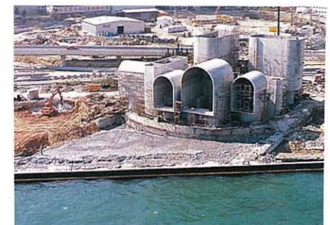
Completed reclamation, Quarry Bay. 鯽魚涌填地竣工
