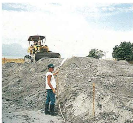
Moisture content adjustment. 含水量調整
