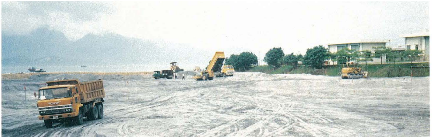
PFA filling operations in progress. 煤灰粉填築施工景象
