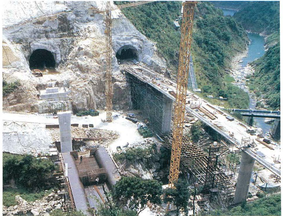
Over 9000 m 3 of PFA concrete were used for the Shing Mun bridges. 城門橋所用煤灰混凝土超過9000立方米
