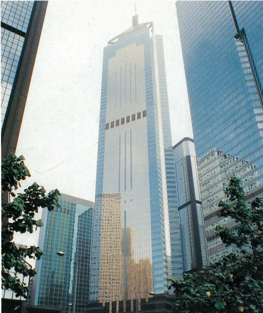
The completed Central Plaza. At 374m it is the world's tallest reinforced concrete building. 眺望完成後的中環廣場，這座 374 米高的建築物是現時世界上最高的鋼筋混凝土大廈。
