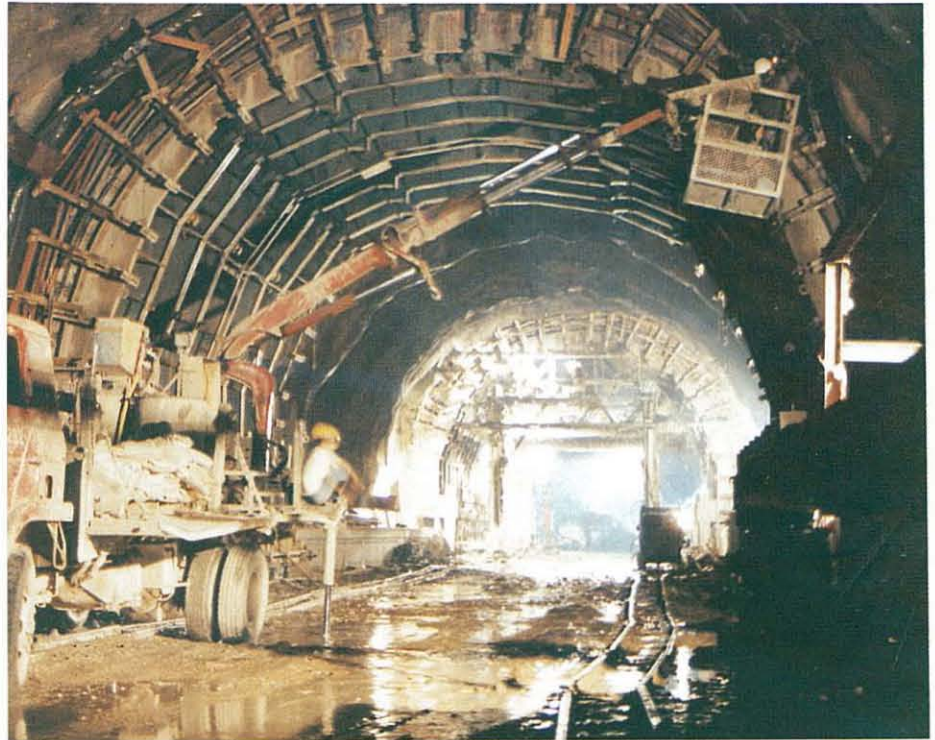
PFA concrete was used in the Shing Mun tunnel linings. 城門隧道襯牆採用煤灰混凝土
