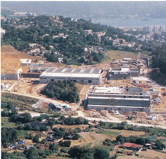
PFA concrete was used in the Pak Kong Water Treatment Works. 北港濾水廠工程採用煤灰混凝土
