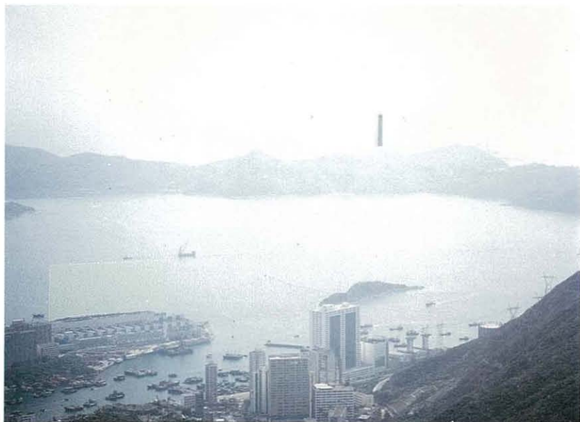
VIEW FROM MAGAZINE GAP ( AP LEI CHAU POWER STATION IN FOREGROUND )
