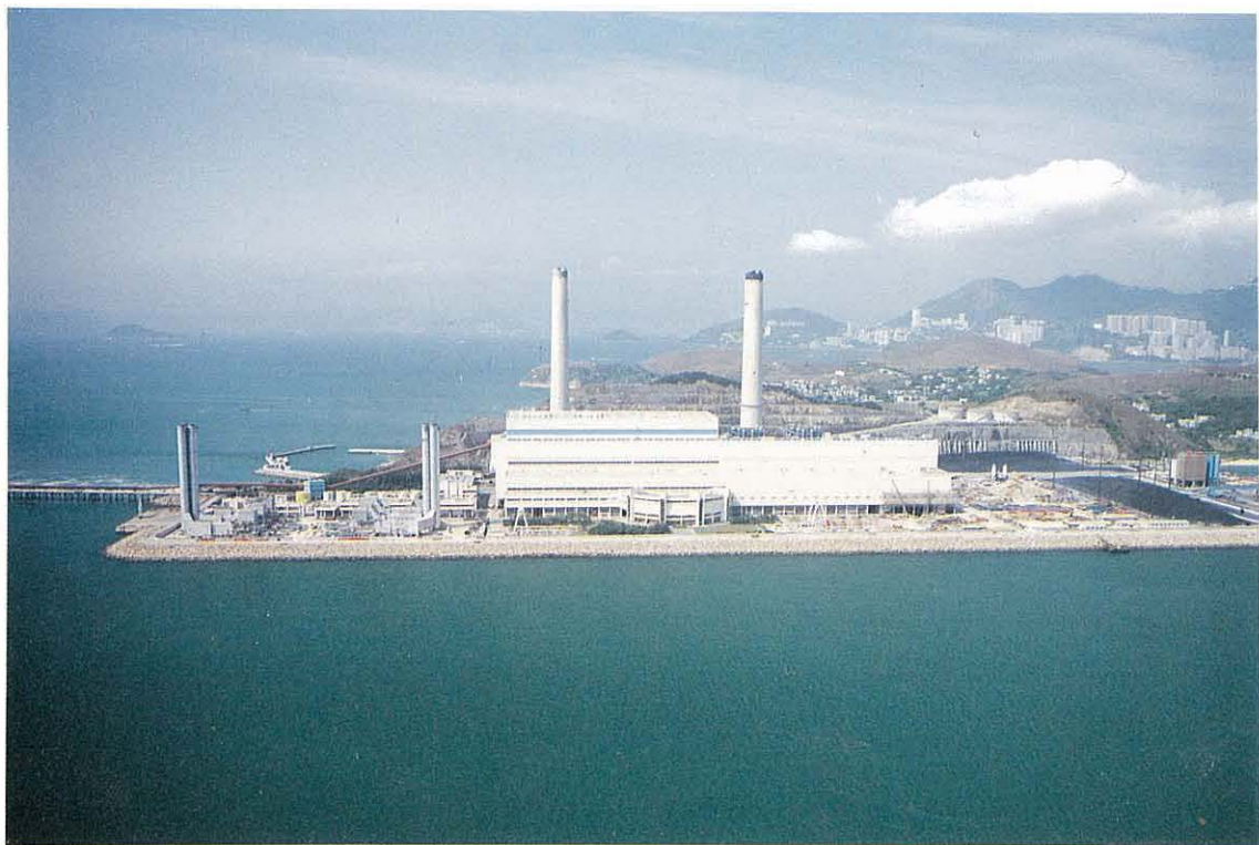
VIEW OF EXISTING POWER STATION
