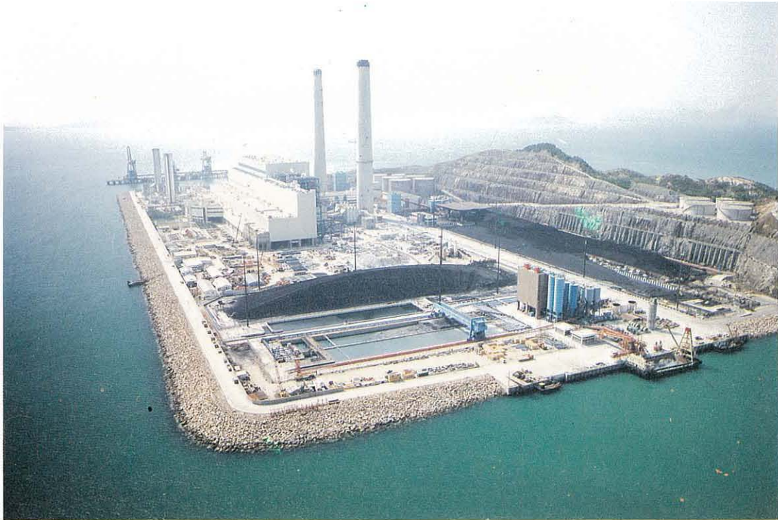
VIEW OF EXISTING POWER STATION
