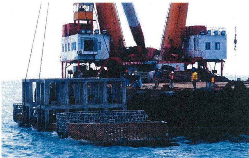
The Agriculture, Fisheries and Conservation Department has implemented an artificial reef programme in phases, which includes reefs within Sha Chau and Lung Kwu Chau Marine Park, and in the MEZ immediately northeast of HKIA.
