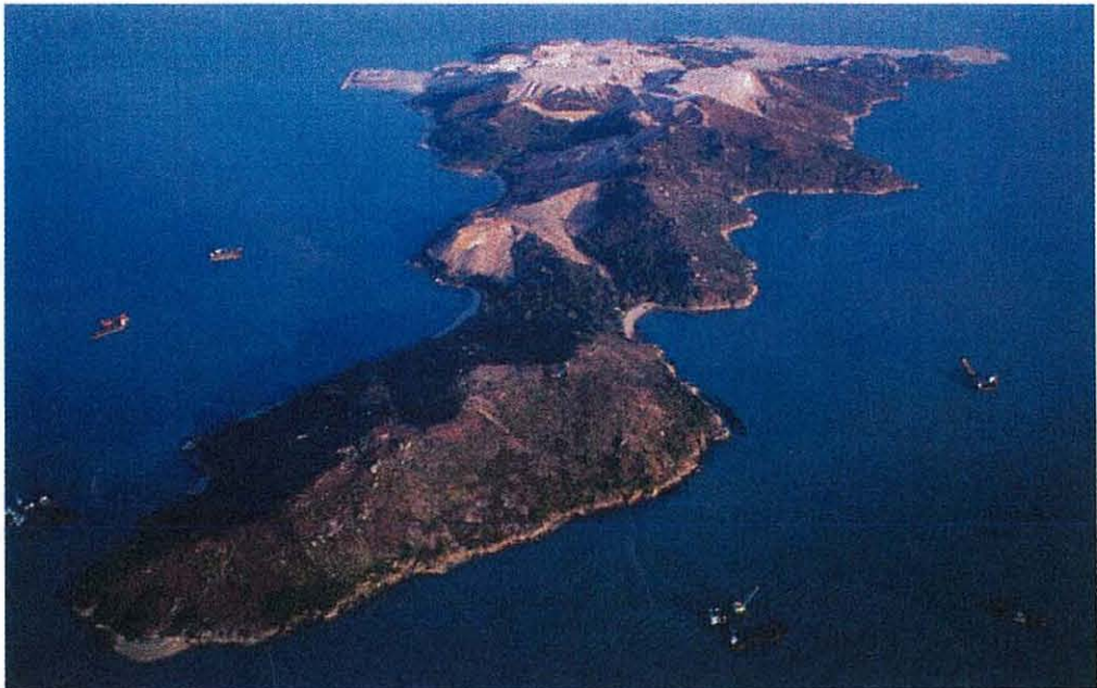
The start of reclamation works at Chek Lap Kok.
