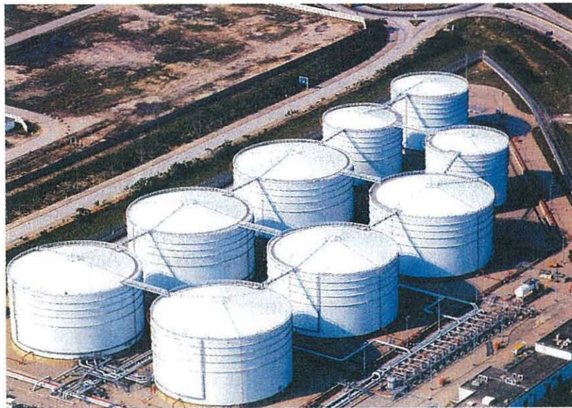
The original Aviation Fuel Tank Farm at HKIA.
