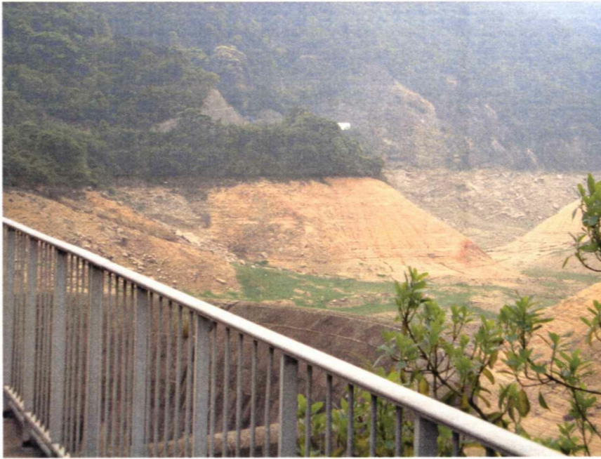
Existing view of Lower Shing Mun Reservoir
