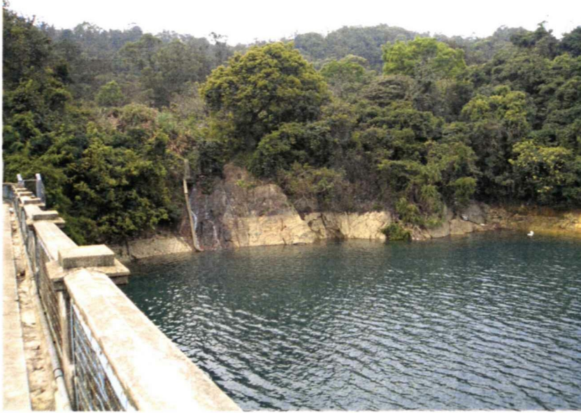
Existing view of Kowloon Byewash Reservoir
