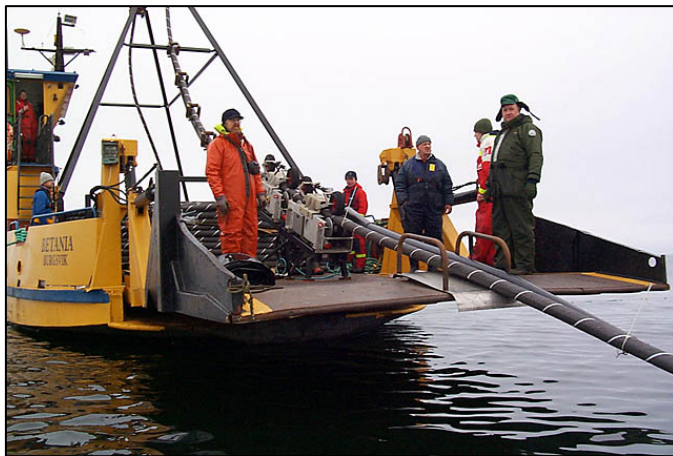
Figure 1.6 – Cable Laying
