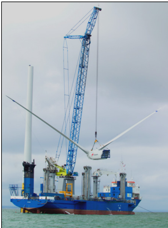
Figure 1.10 – Turbine Installation*
