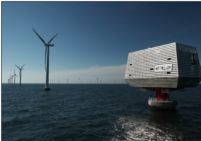
Figure 1.7 – Offshore Transformer Platform*
