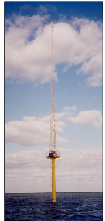
Figure 1.8 Offshore wind monitoring mast
