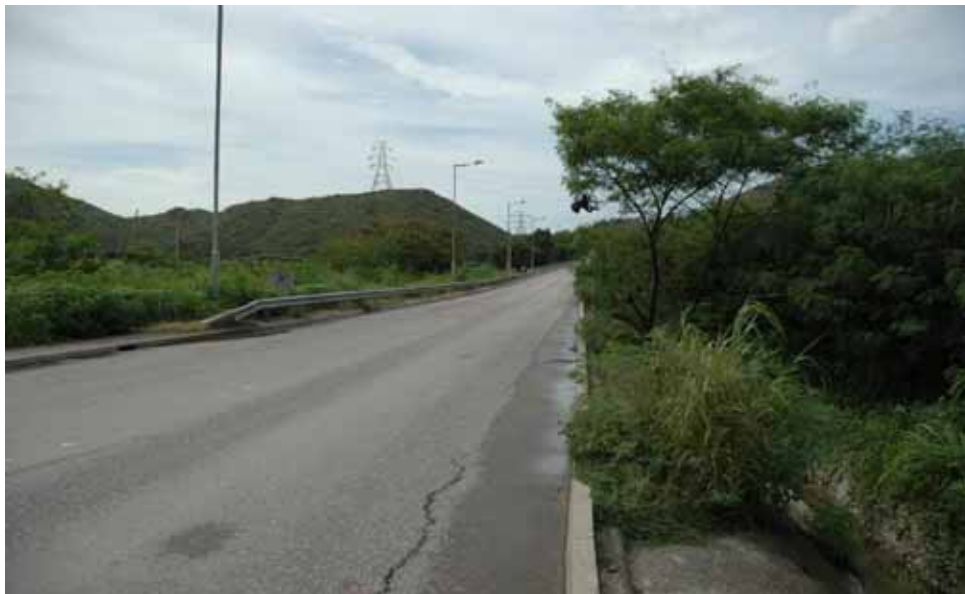
Lung Kwu Tan Road along the site boundary west (View towards north)
