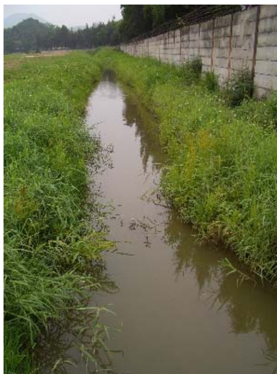
Plate 2 : Site Photo for the Drainage Ditch of Wo Shang Wai
