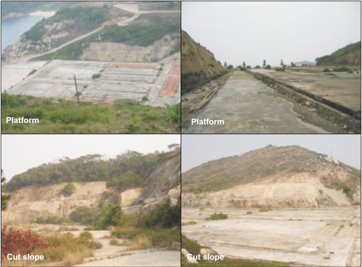
Figure 2.4d Existing Condition of South Soko (Photographs Taken in 2004)
