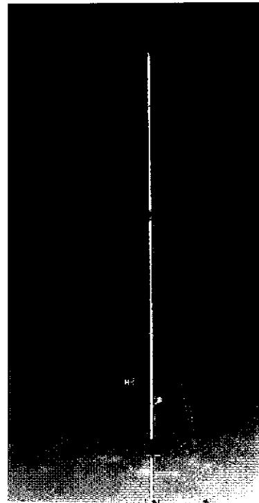
Figure 21. 20m wind monitoring tower.
