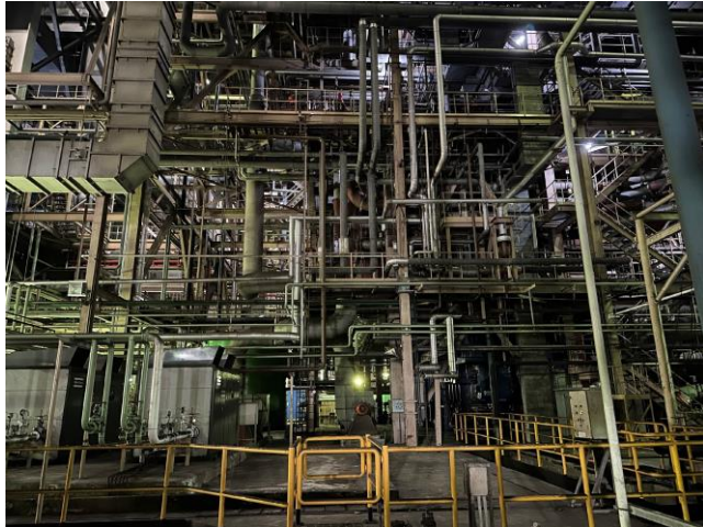
Photo 1: Overall view inside the Main Station Building
