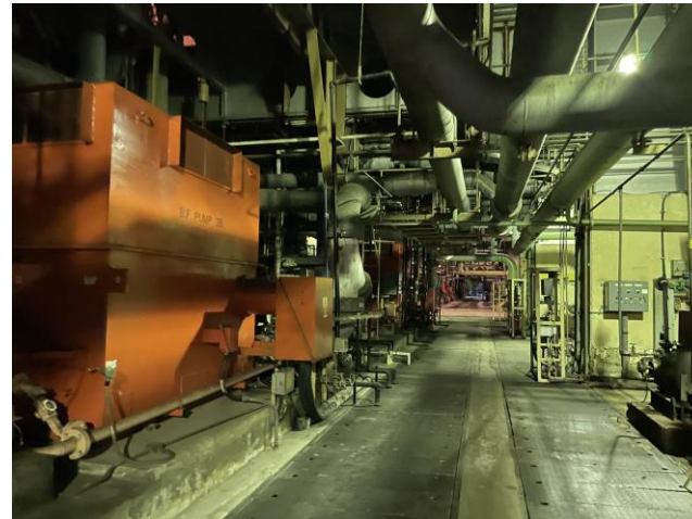
Photo 5: Overall view inside the Main Station Building
