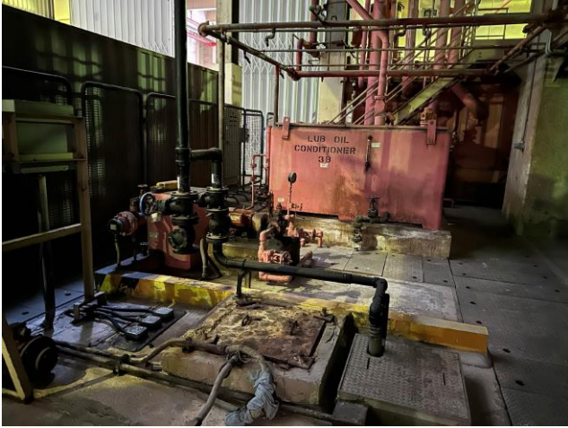
Photo 31: Lubrication oil, oil pumps and sump pit at L3 with oil stains observed
