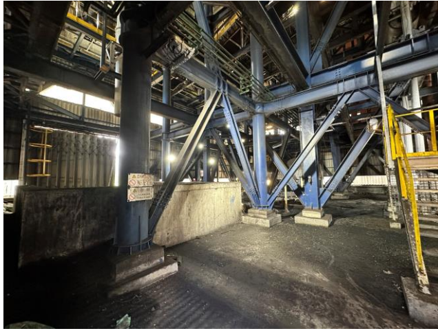
Photo 91: Inside of Junction Tower T16, coal pieces and mixture of coal residuals on ground
