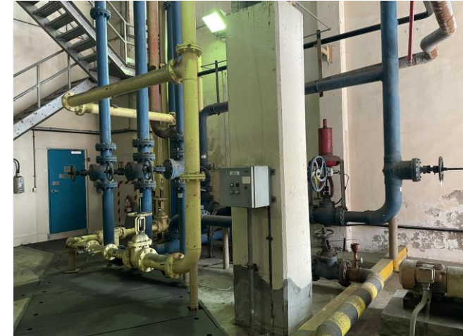
Photo 24: Oil transfer pump
