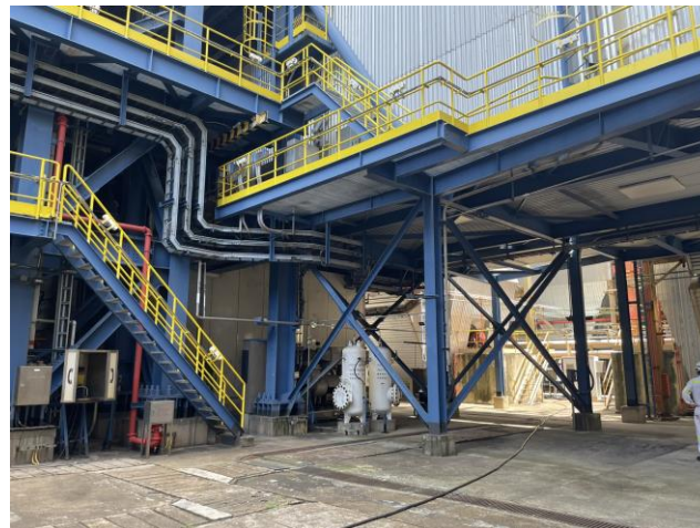
Photo 65: Structures of the Flue Gas Desulphurisation (FGD) plant
