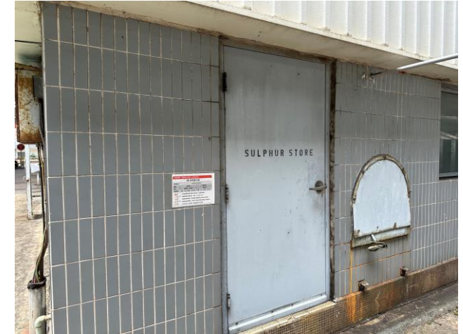
Photo 81: Storage of Sulphur solid
