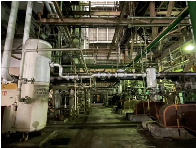
Photo 4: Overall view inside the Main Station Building
