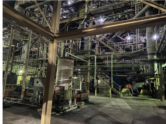
Photo 2: Overall view inside the Main Station Building
