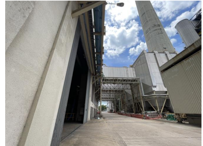
Photo 93: Overview of the Precipitation Road
