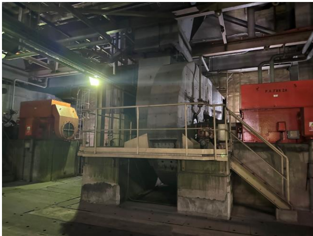
Photo 40: Primary air fan units
