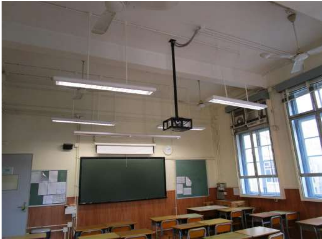
General View No. GV45 Description General view of typical classroom
