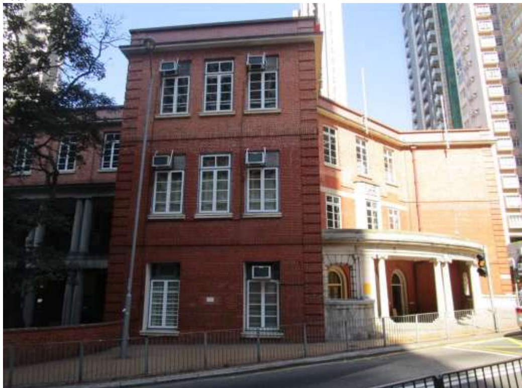
General View No. GV2 Description General view of east wing, south elevation
