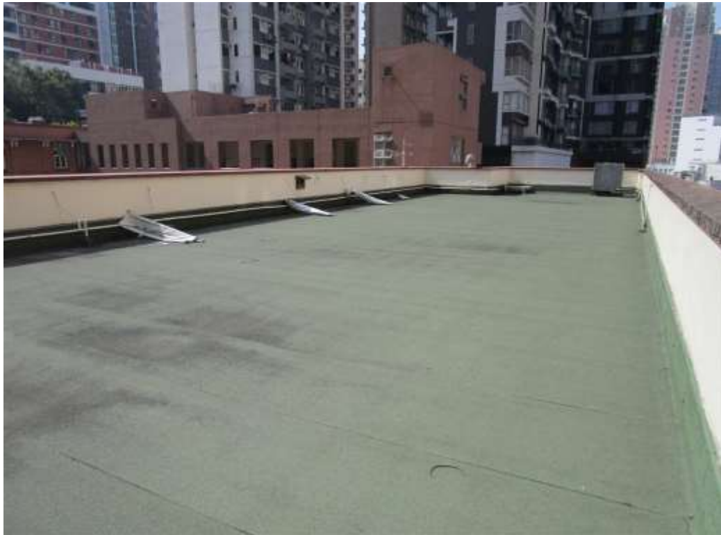
General View No. GV21 Description General view of north wing's roof
