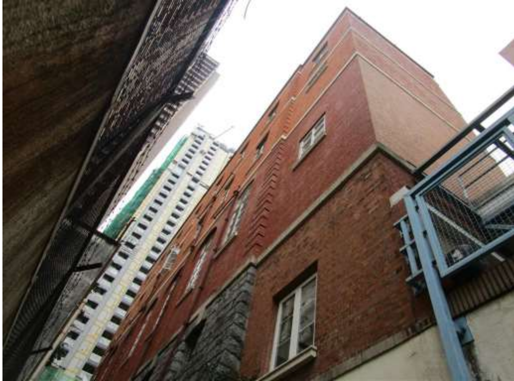
General View No. GV47 Description General view of north wing, north elevation
