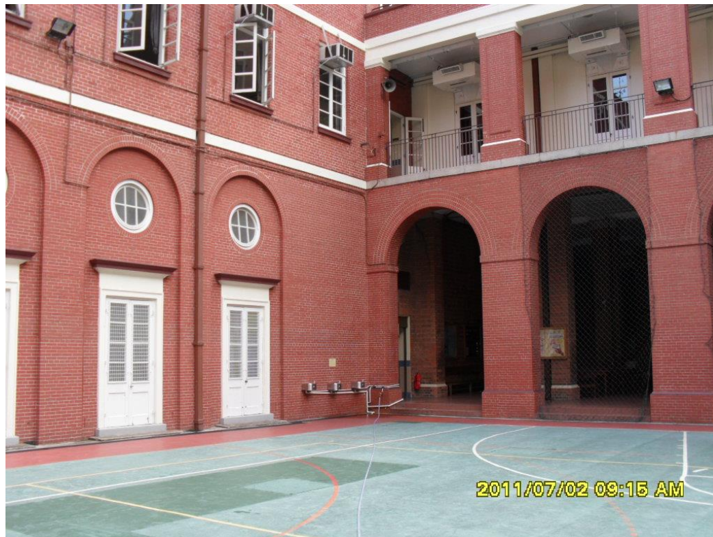
Plate 10: General View of the Feature Crest at the Eastern Portion
