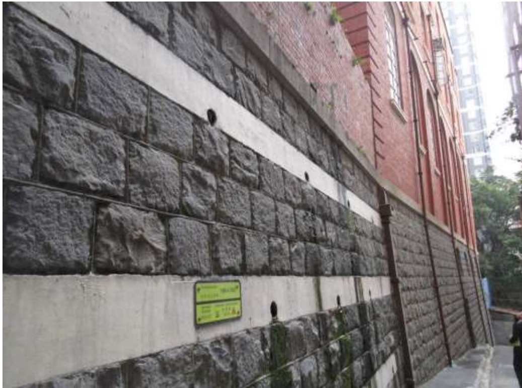
General View No. GV13 Description General view of north retaining wall
