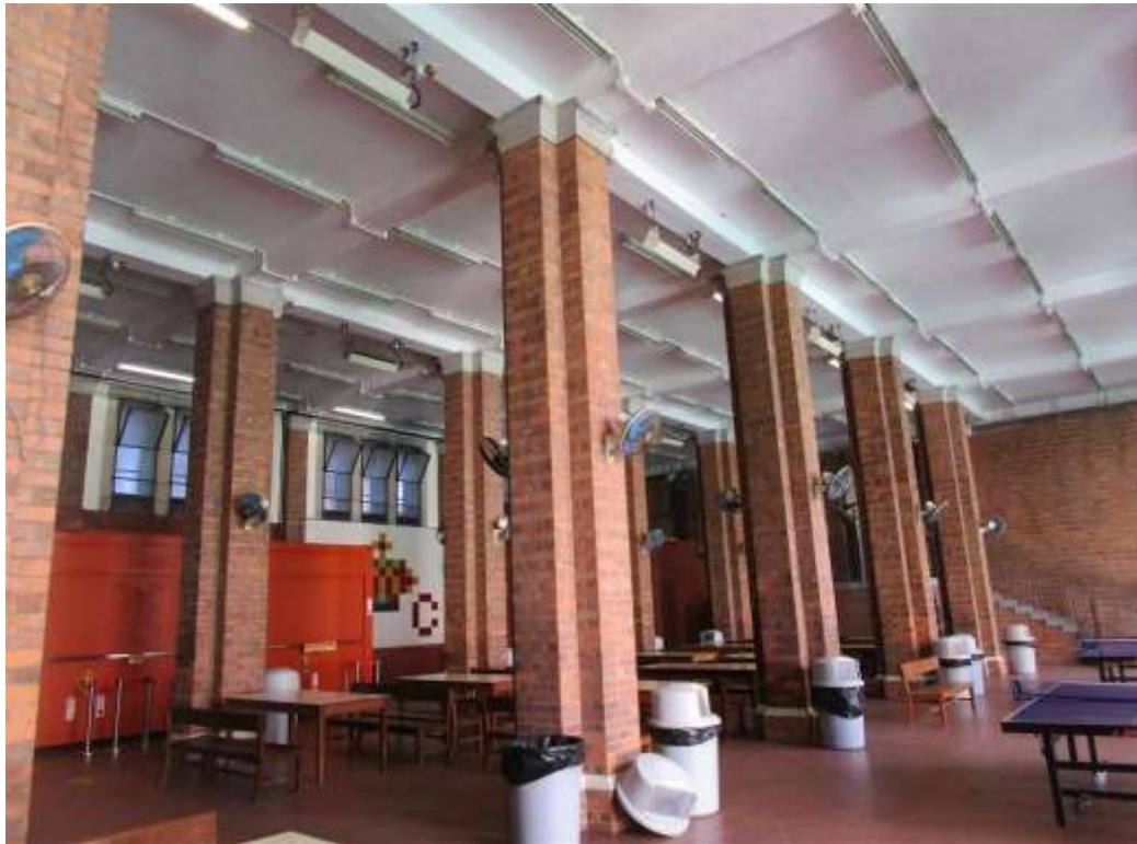
General View No. GV8 Description General view of east wing, canteen
