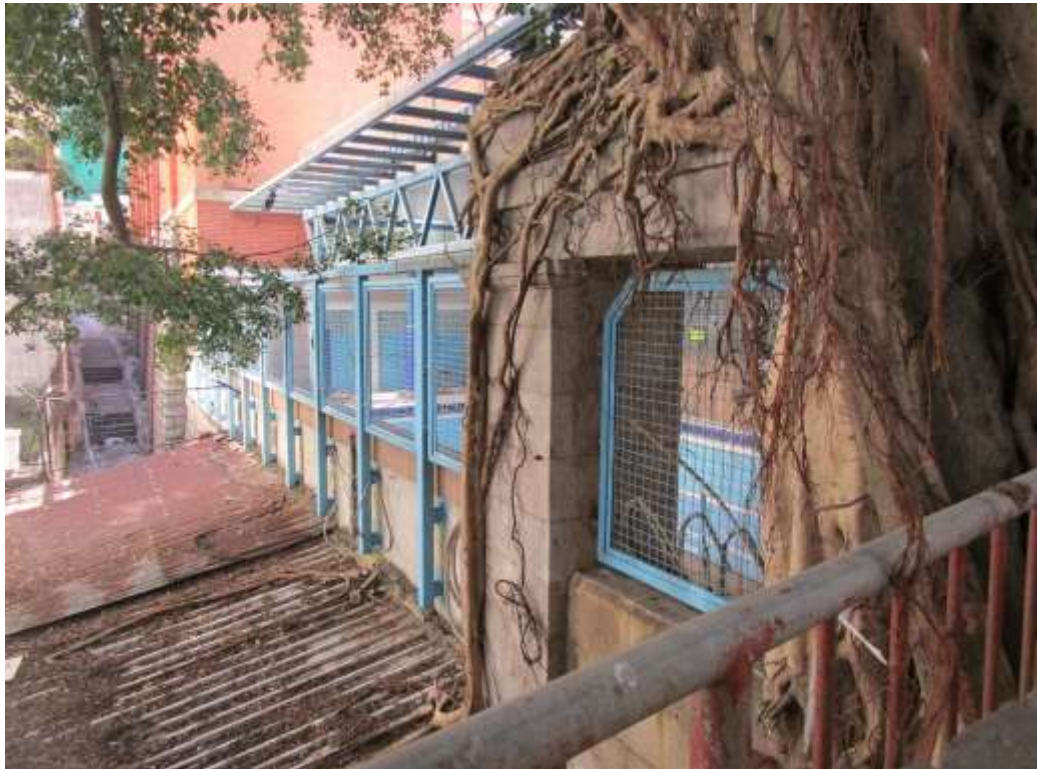
General View No. GV12
