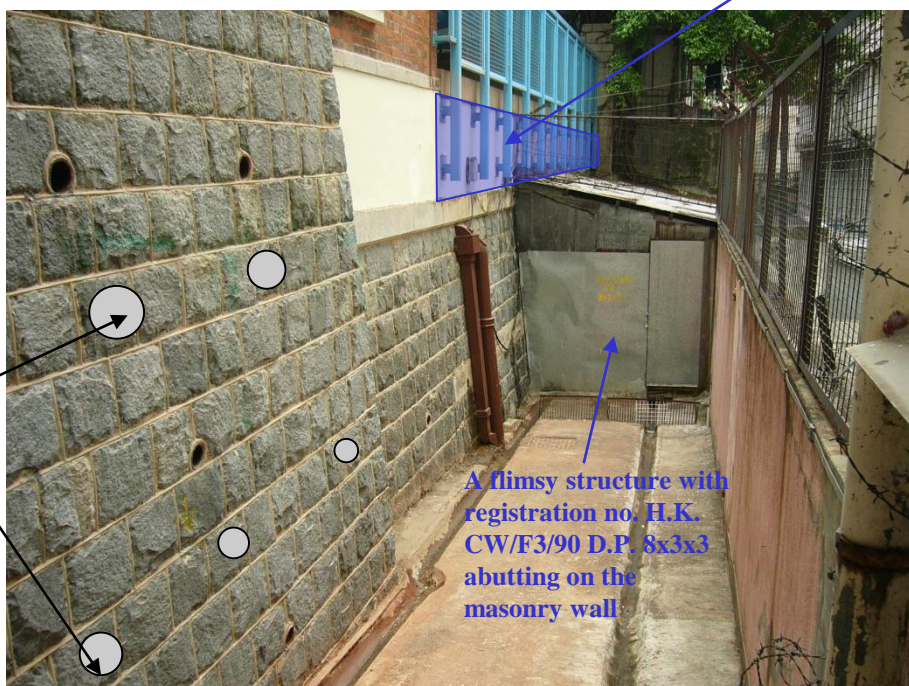
Proposed soil nails at the western portion
