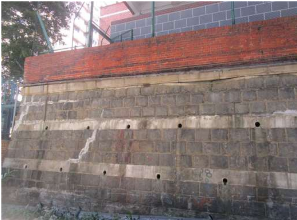
General View No. GV42
