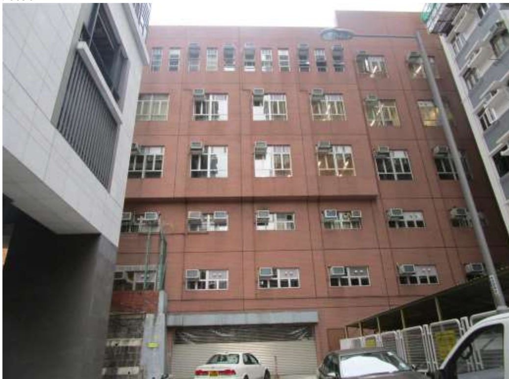
General View No. GV50 Description General view of west wing, west elevation
