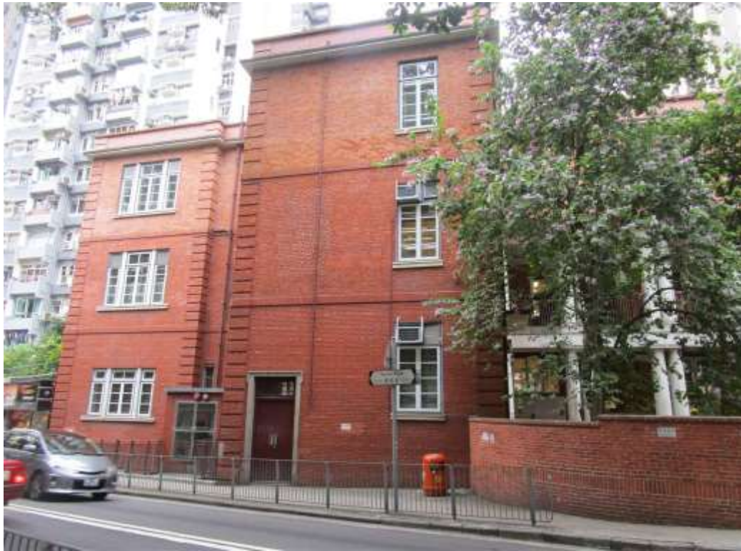
General View No. GV53
