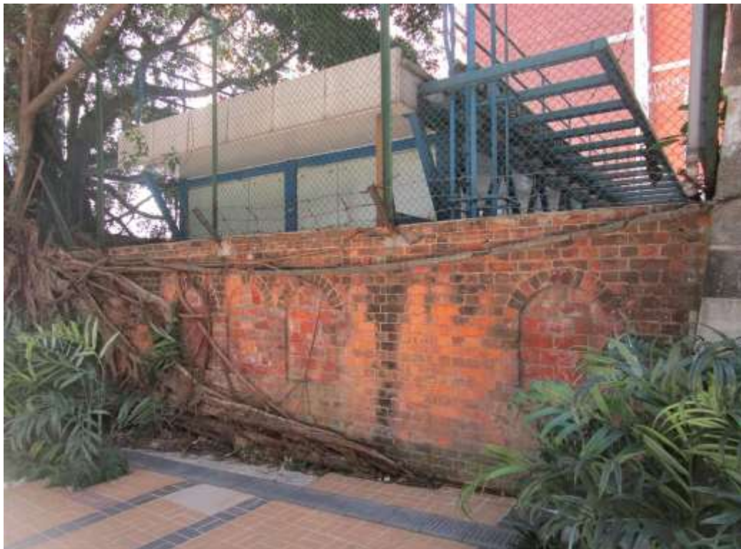
General View No. GV26
