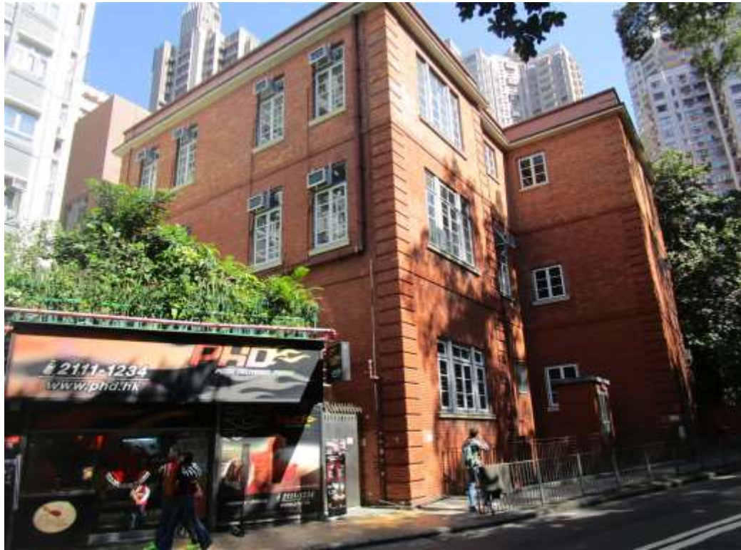
General View No. GV35 Description General view of south wing, west elevation viewed from south Photo No. 0036
