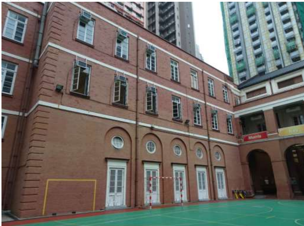
General View No. GV20 Description General view of north wing, south elevation
