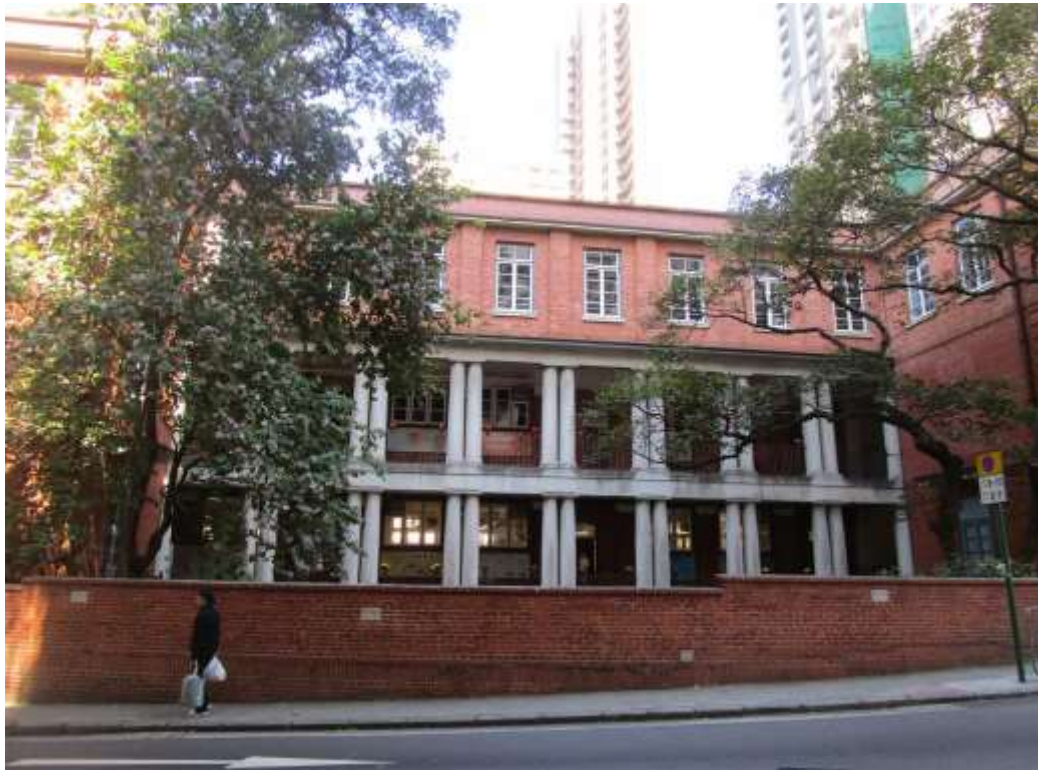
General View No. GV33 Description General view of south wing, south elevation
