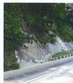
Before slope upgrading works
