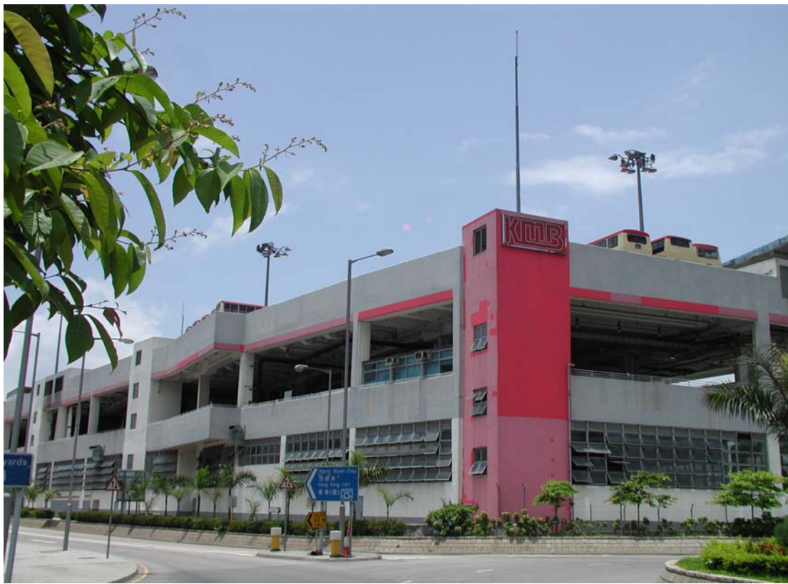
Kowloon Motor Bus Depot Southwest of the Subject Site
