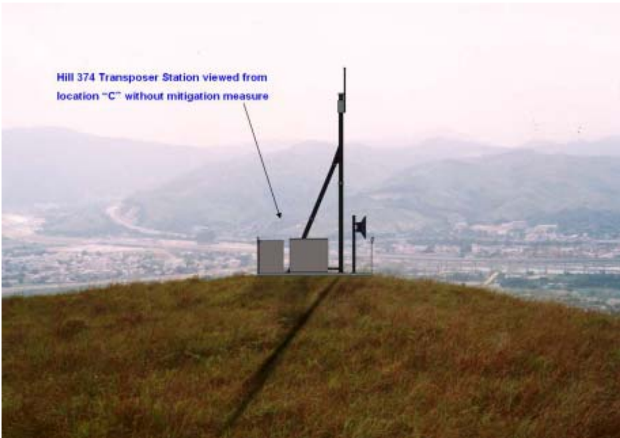
Figure 15: Proposed Hill 374 Transposer Station viewed from location "C" without mitigation measures
