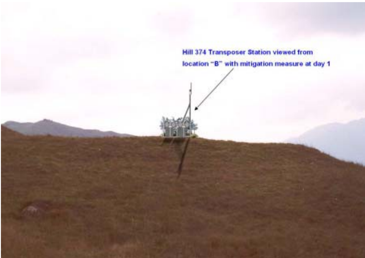
Figure 13: Proposed Hill 374 Transposer Station viewed from location "B" with mitigation measures at day 1 of the operation stage
