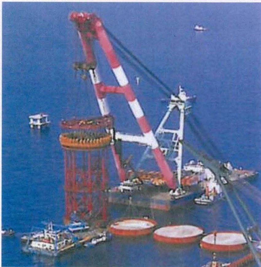
Marine Plant for Caissons Installation 安裝沉箱工程的海上設備
