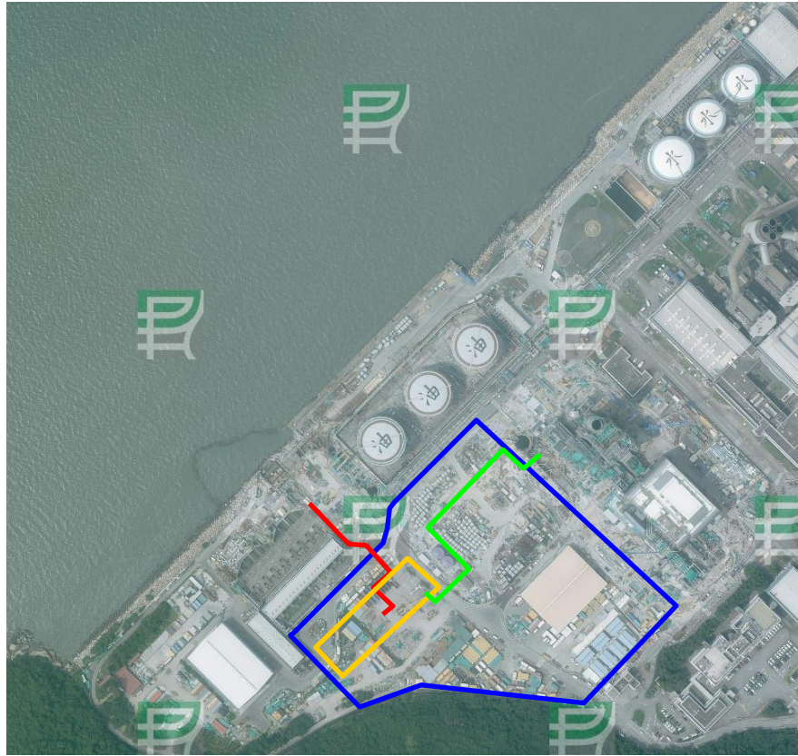
Year 2019 (ref: E063237C, height: 6,900m) No significant changes were observed compared to 2018. No construction / industrial activities were observed.
