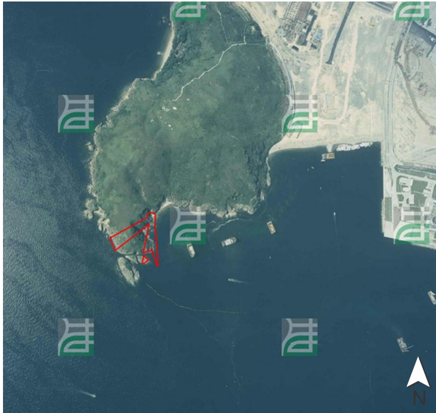
Year 1996: No significant change was observed at the cable landing site. Reclamation of TKO137 Fill Bank was in progress.
