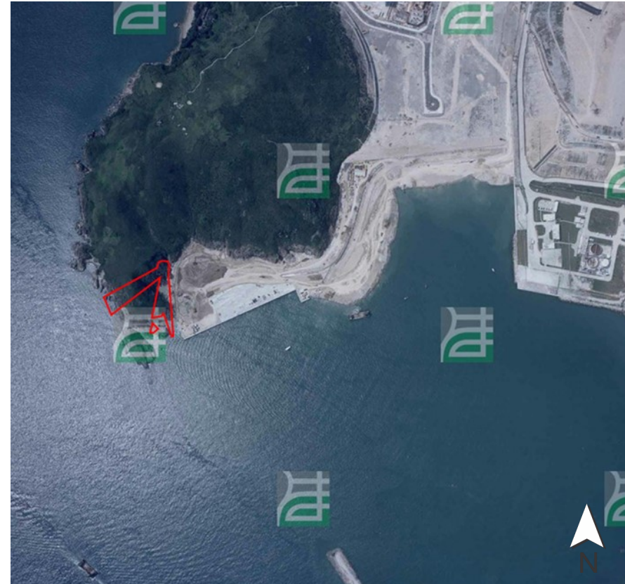
Year 1997: The cable landing site was mainly comprised of island and sea. Reclamation of area near the cable landing site was in progress.
