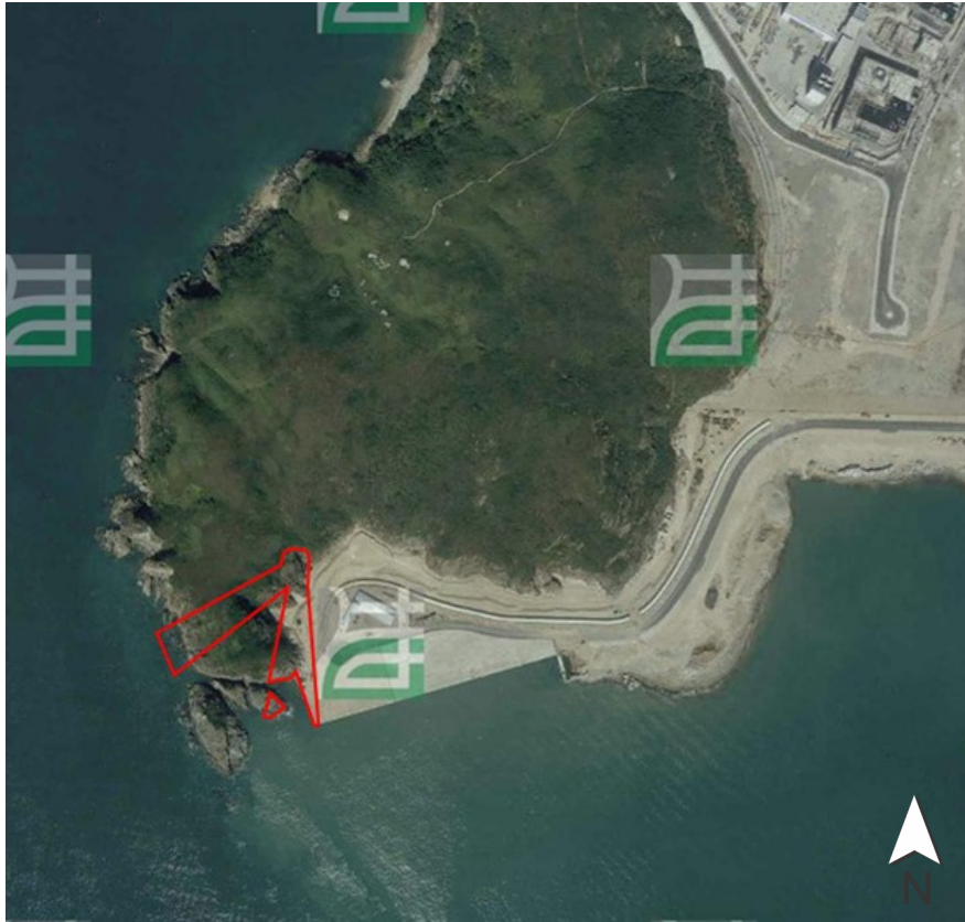
Year 1997: No significant change was observed at the cable landing site. Reclamation of TKO137 Fill Bank was in progress.
