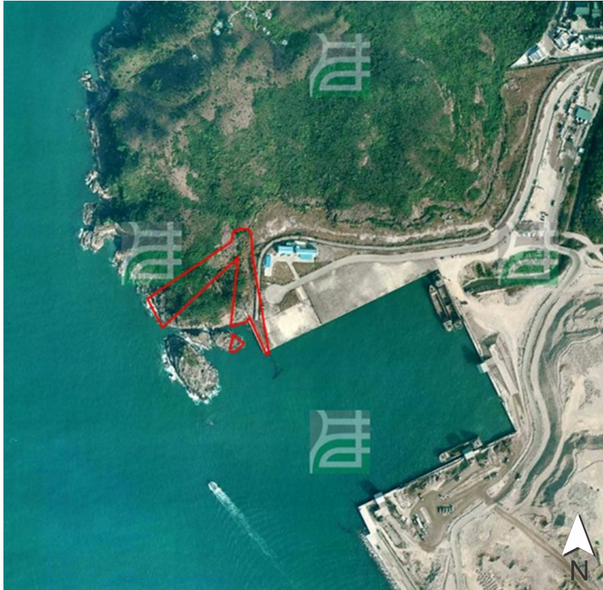
Year 2007: No significant change was observed at the cable landing site.
