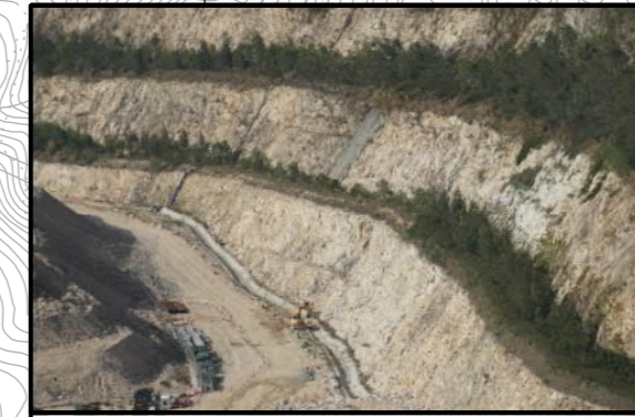
PHOTO 1001: NORTHERN ROCK SLOPE AT ARO SITE DATE TAKEN: 21 MARCH 2018
