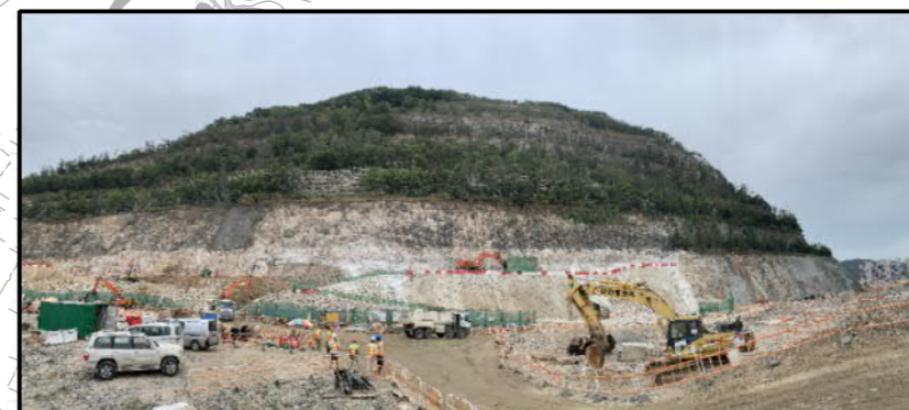
PHOTO 1003: NORTHERN ROCK SLOPE AT ARO SITE DATE TAKEN: 13 NOVEMBER 2020
