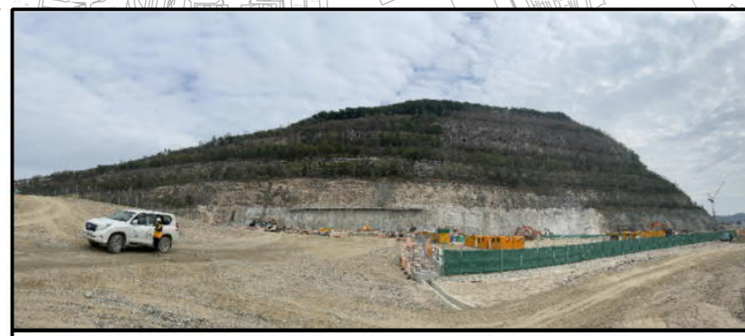
PHOTO1004: NORTHERN ROCK SLOPE AT ARO SITE DATE TAKEN: 19 JANUARY 2022
