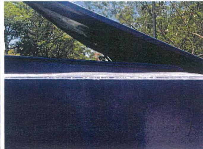
Photo 4 – Sealing of Top Cover
