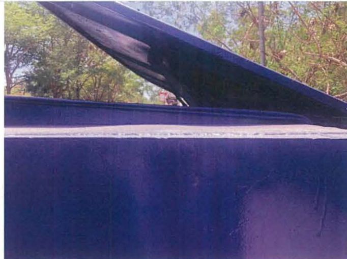
Photo 4 – Sealing of Top Cover
