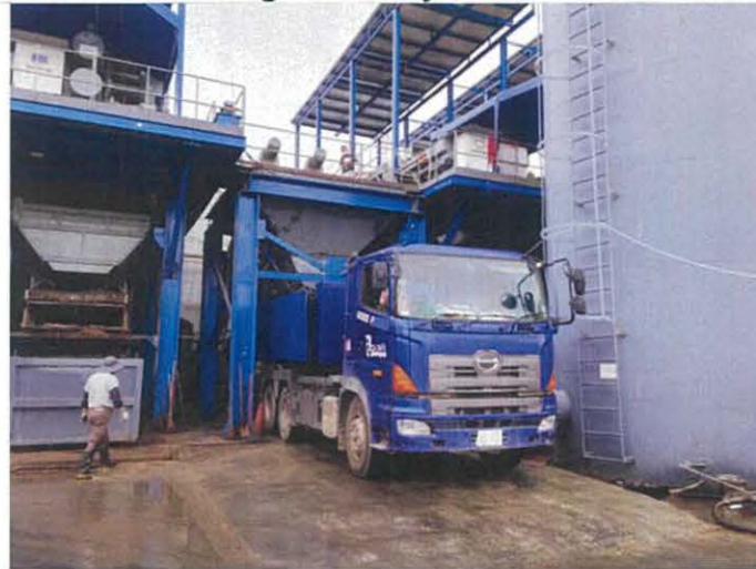
Photo 2 – Loading of GTW Sludge to Enclosed and Water-tight Container Truck at the Waste Cooking Oil Recycling Plant
