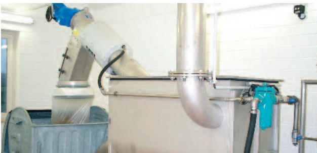
Tank-mounted HUBER Rotary Drum Fine Screen ROTAMAT®...
