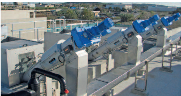
3 ROTAMAT® STAR units size 1000 with 1.5 mm perforation protecting the downstream membrane plant
