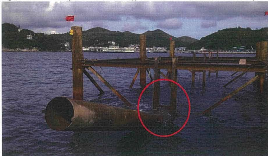
Figure 2.2 Photo of Similar Steel Scaffold Constructed under a Past Project
