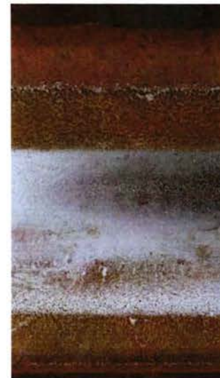
Running Surface of Near Rail
