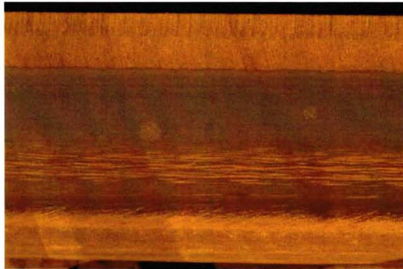
Running Surface of Near Rail
