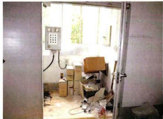
Photo 6 Overview of the Incinerator Room
