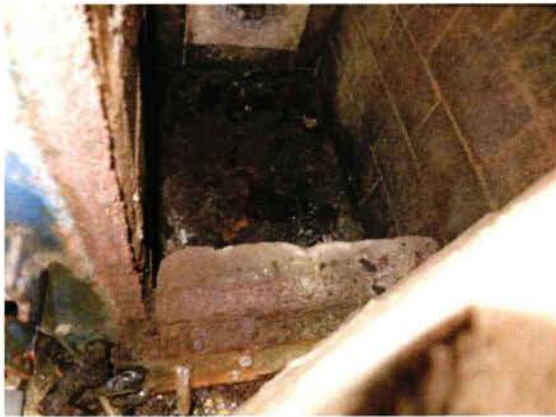
Photo 3 Residual bottom ash at the bottom of the combustion chamber
