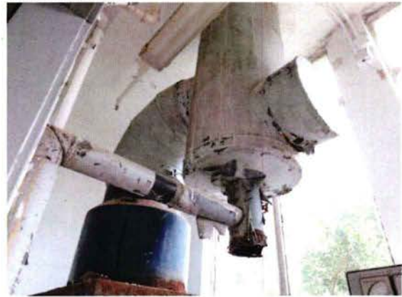
Photo 4 Chimney of the incinerator
