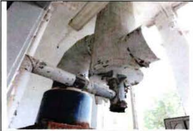
Items (1.3) and (1.4) Chimney
