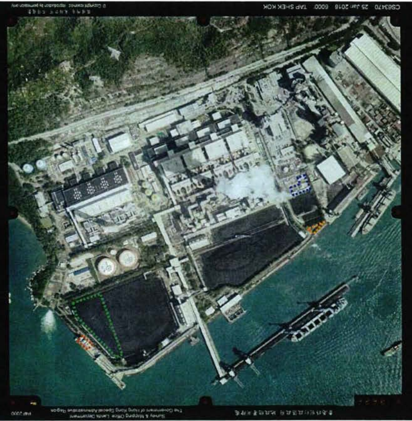
Year 2016 (ref: CS63470 height: 6,000ft) Works Area A: Contractor Village – No significant changes were observed compared to 2013. Works Area B: South of Lagoon No.1 – No significant changes were observed compared to 2013. Works Area C: West Coal Stockyard – No significant changes were observed compared to 2013. Works Area D: Existing Silos along Sea Bank Road West – No significant changes were observed compared to 2013.
