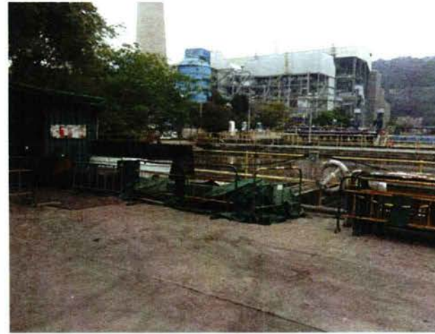
Photo 6: Area next to Lagoon No. 1 is concrete paved and stored with construction materials.
