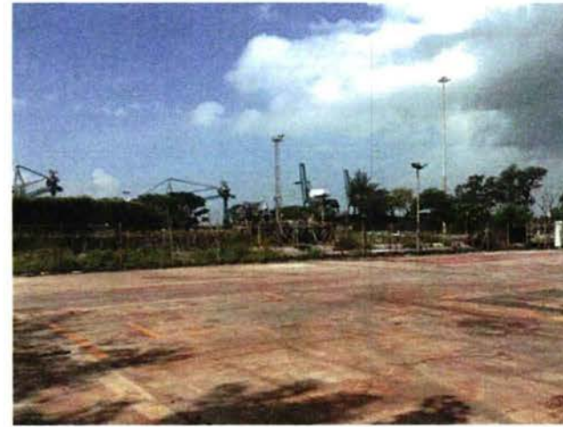
Photo 2: Contractor Village area is concrete paved.
