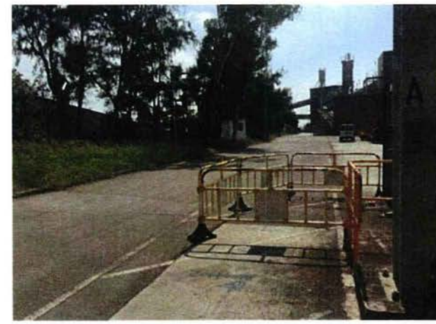
Photo 8: Sea bank road west.
