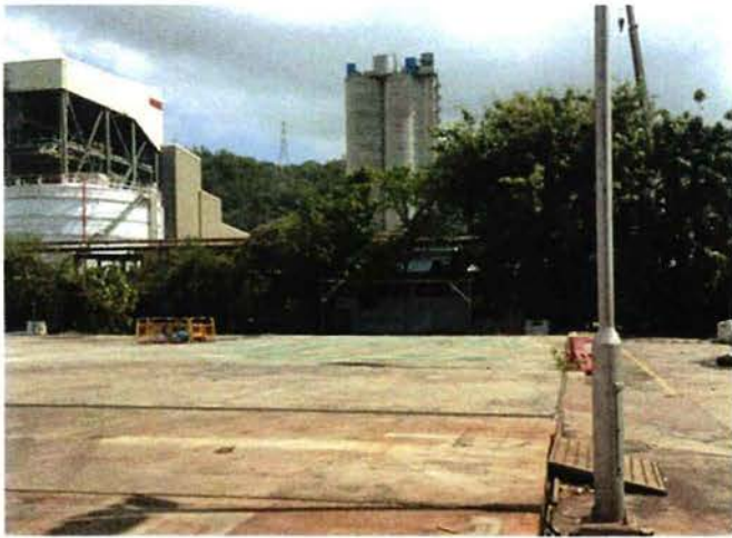
Photo 1: Contractor Village area is concrete paved.
