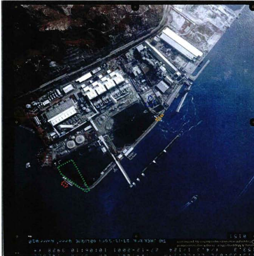
Year 2001 (ref: RW00428, height: 4,000ft) Works Area A: Contractor Village – The temporary offices buildings observed in 1996 were replaced with temporary structures and material storage. Works Area B: South of Lagoon No.1 – Small amount of material storage were observed. Works Area C: West Coal Stockyard – No significant changes were observed compared to 1996. Works Area D: Existing Silos along Sea Bank Road West – No significant changes were observed compared to 1996
