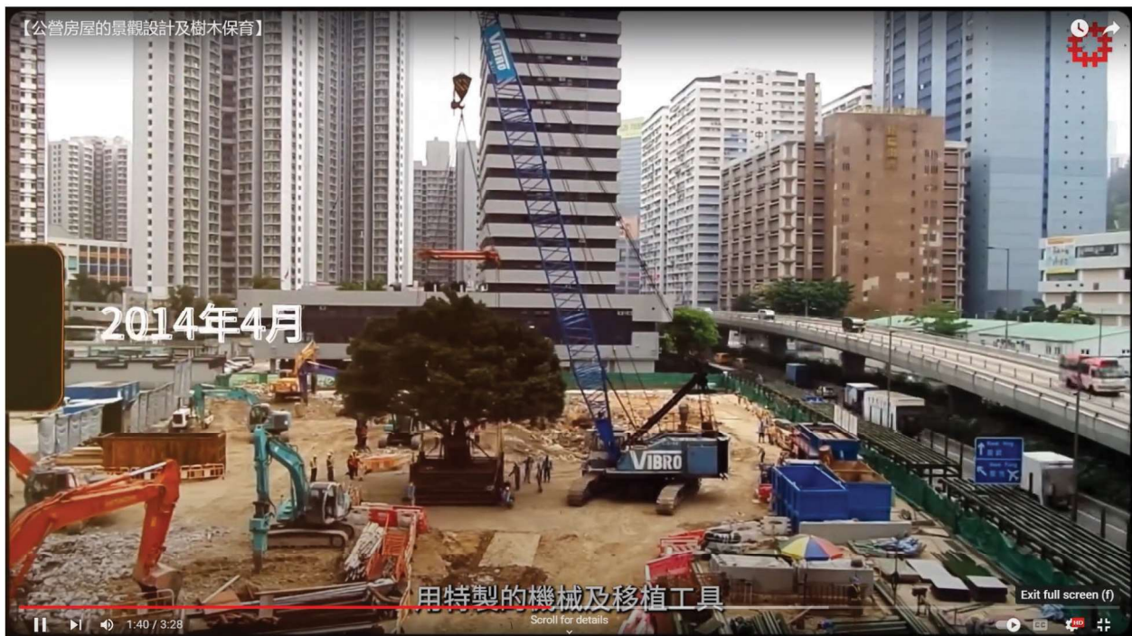
Figure 5I – Screen clipped from the video recording the tree transplanting in Kwai Tsui Estate
