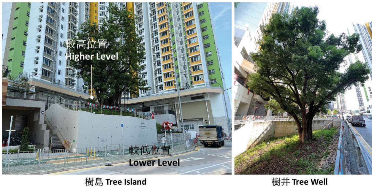
Figure 5E – Example of tree island and tree well for the preserved tree to cater for the level difference of the development and the ground level of the preserved tree (Photos taken from the housing development in Queen’s Hill)
