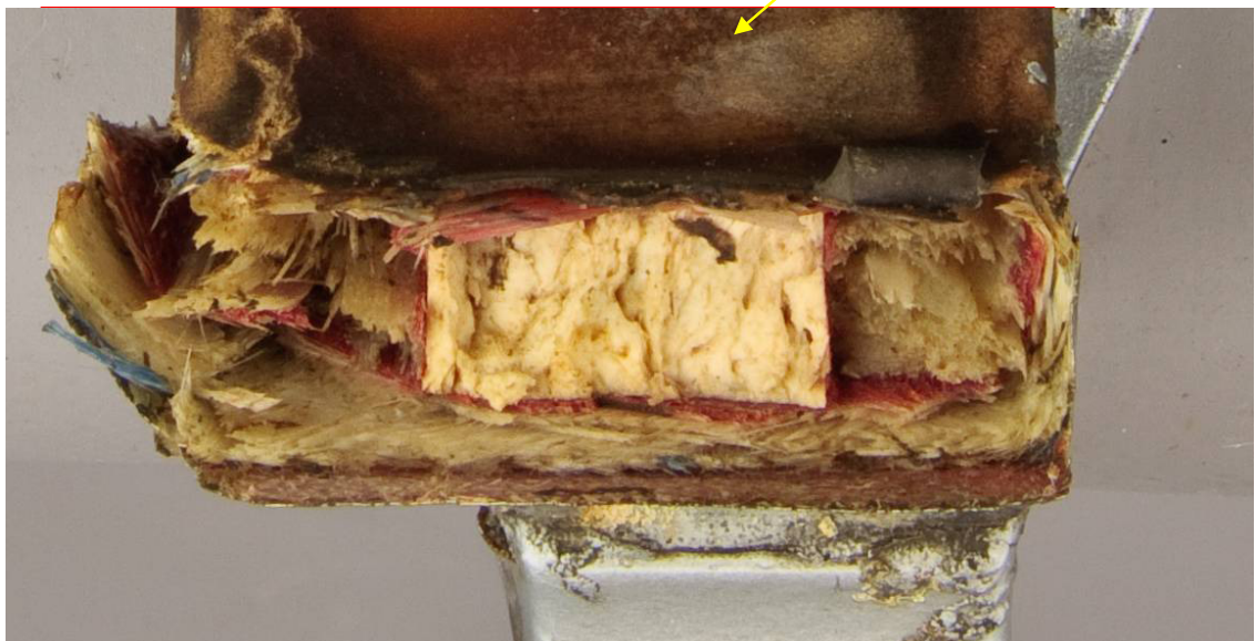
Figure 56 - Photographs showing a plan view of the fractured root area of the White blade after removal of the elastomeric bearing, with detail of the fractured trailing edge arm shown in the bottom insert image
