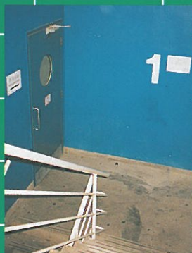
Staircase and fire door
