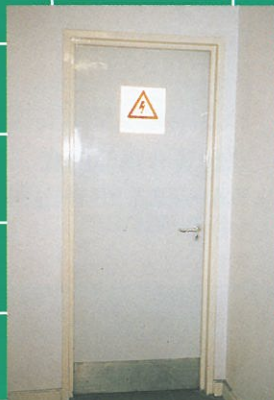
Special hazard room
