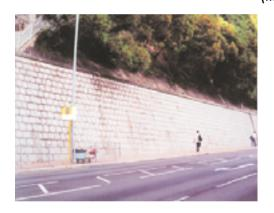
(iii) Most slope or retaining wall failures are associated with water. Slopes adjoining water courses have to be more frequently monitored. Prolonged rainfall, blocked subsoil drainage, broken surface channels, deteriorated surface coverings, surge of ground water table are contributing factors to slope or retaining wall failure.
