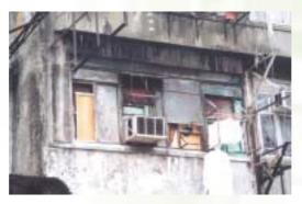
shorten their life-span. When excessive forces are applied to operate such windows or when they are subject to wind load, distortion or dislodgement of the window sashes or even the frame may result, causing fatal or serious injuries to the public.
