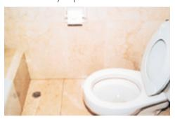
habit, the waterproofing system of the floor is put to test. Should the cause be identified as water spilled on to the floor, it is always advisable to reconstruct the entire waterproofing layer instead of patch repair.
