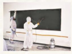
asbestos consultant to carry out an investigation, suggest asbestos abatement plan and / or asbestos management plan if asbestos is found, and supervise the abatement work. All the removal work of asbestos containing materials should be done by a qualified contractor.
