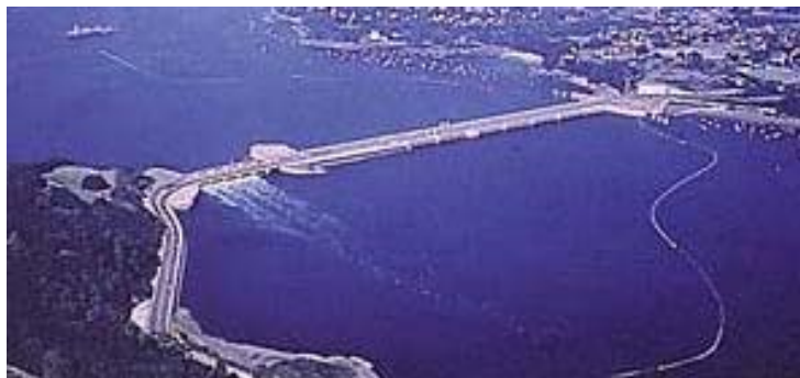
Figure 9-7: La Rance 240 MW Station in France (Source: Australian Greenhouse Office)
